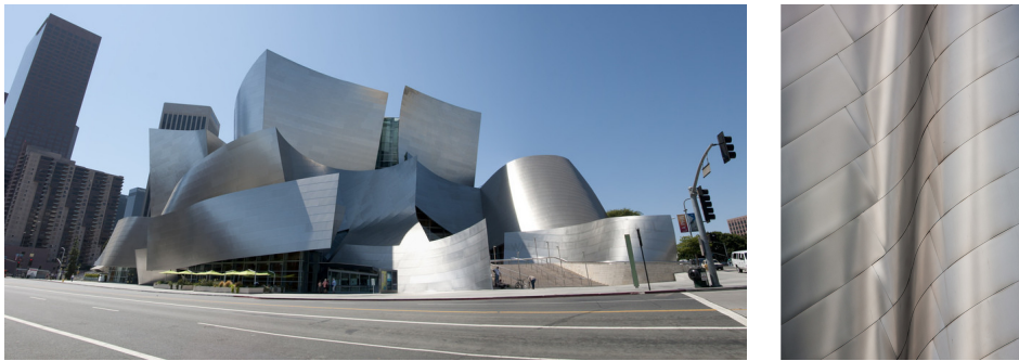
Figure 1.1: Walt Disney concert hall and the steel panels.
