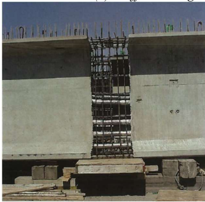
(b) In-span splice
