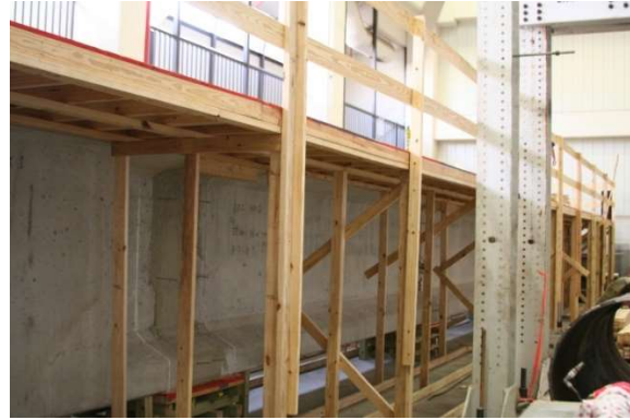
(b) North Side Formwork
