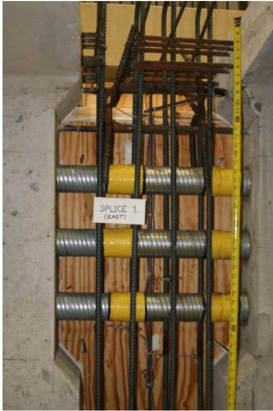
(a) Splice 1 (End)
