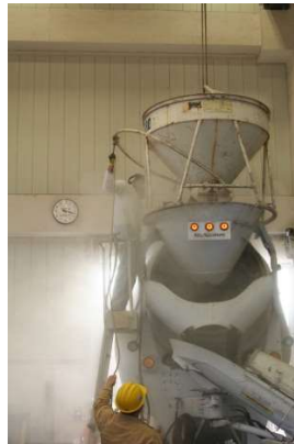
(b) Adding Cement to Truck
