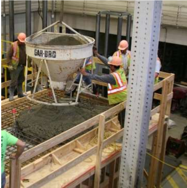
(a) Casting the Deck
