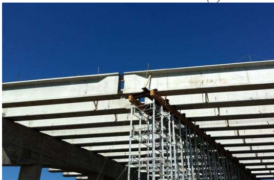
(c) In-span splices in the back span on shoring towers
