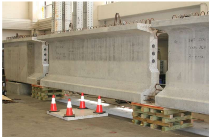
(b) Side View - Girder Alignment
