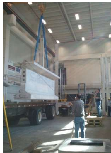
(b) Placing Girder Segments
