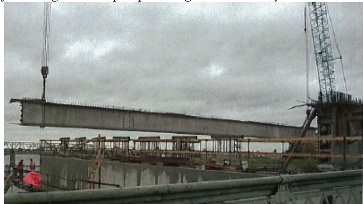
(c) Erection of entire span
