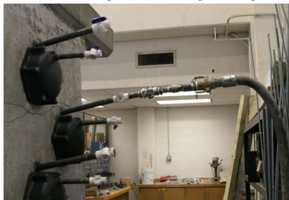
(e) Grouting Ducts Using Air Pressure
