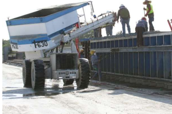
(b) Casting Concrete Transported from Batch Plant
