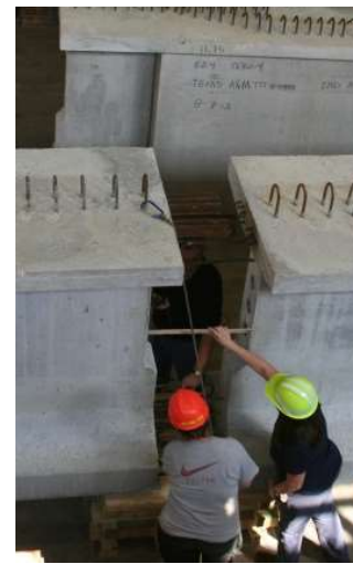
(c) Verifying Segment Spacing and Placement
