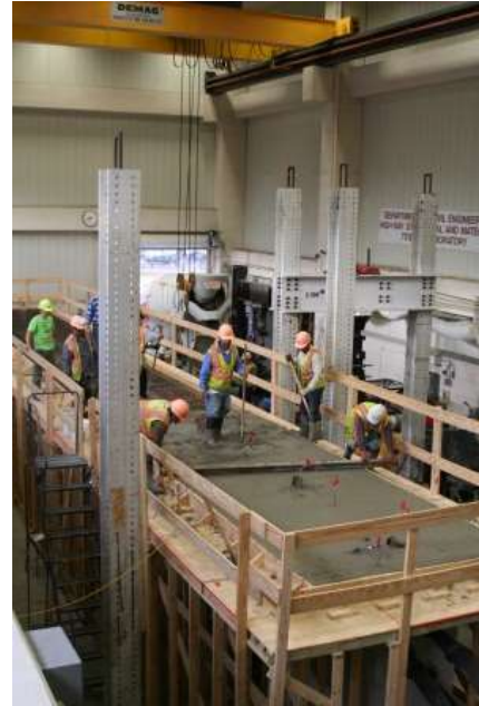
(b) Finishing the Deck
