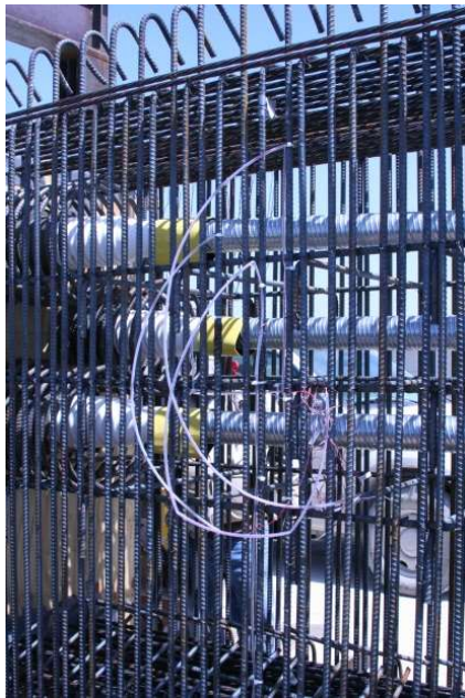
(c) Protecting Gage Wires
