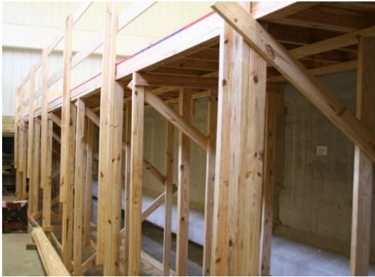
(a) South Side Formwork
