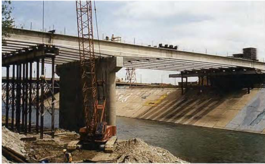
(a) Shoring towers provided in the back-span in partially shored construction
