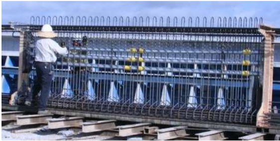
(a) Installing Reinforcement
