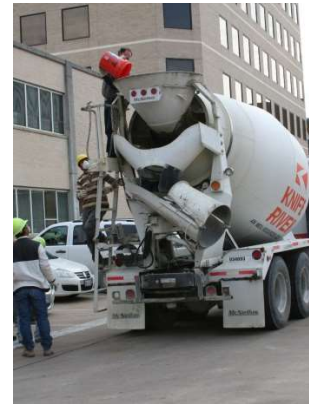
(c) Adding Admixture and Water to Truck
