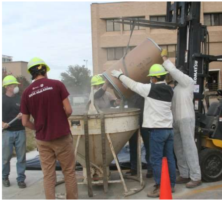
(a) Measuring Cement into Hopper
