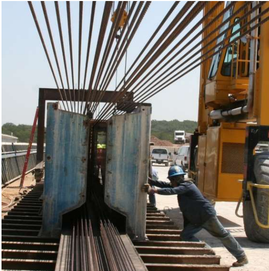
(a) Installing Formwork
