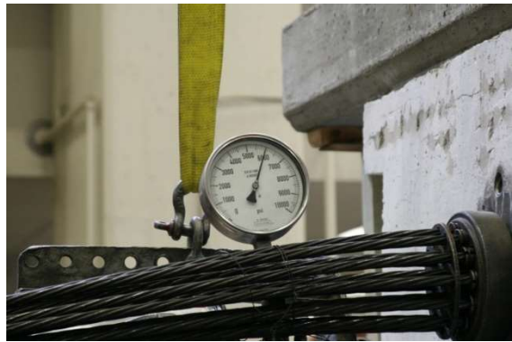
(c) Measuring Pressure during Stressing
