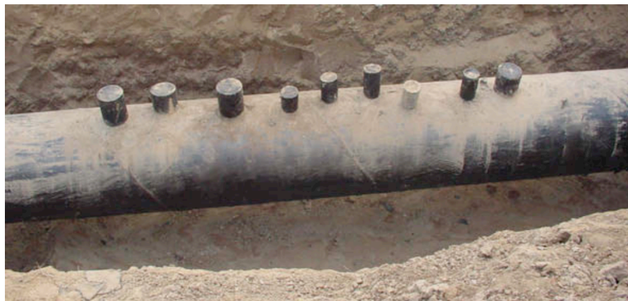
Figure 9. 5m-long drilled pipeline segment with 9 holes [37].
