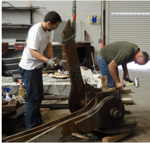
Figure 3-1 – Eyebar Joint Dismantling
