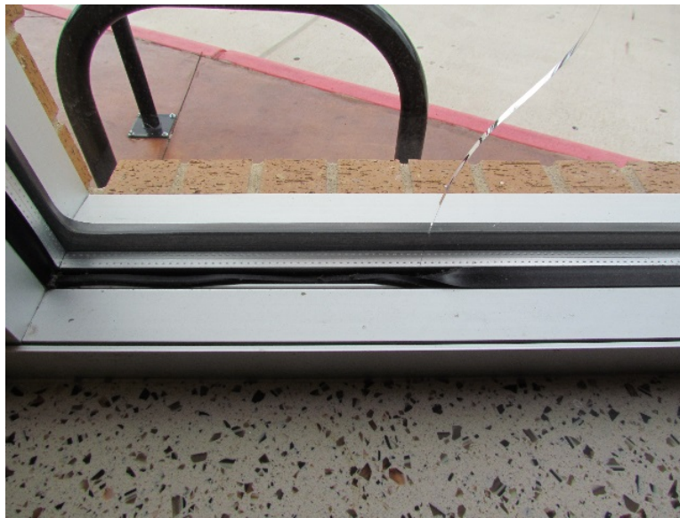
Fig. 8. Glass Plate Breakage due to Thermal Stress
