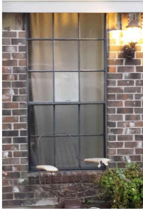
Fig. 14. Residential Window with Different Solar Absorptances
