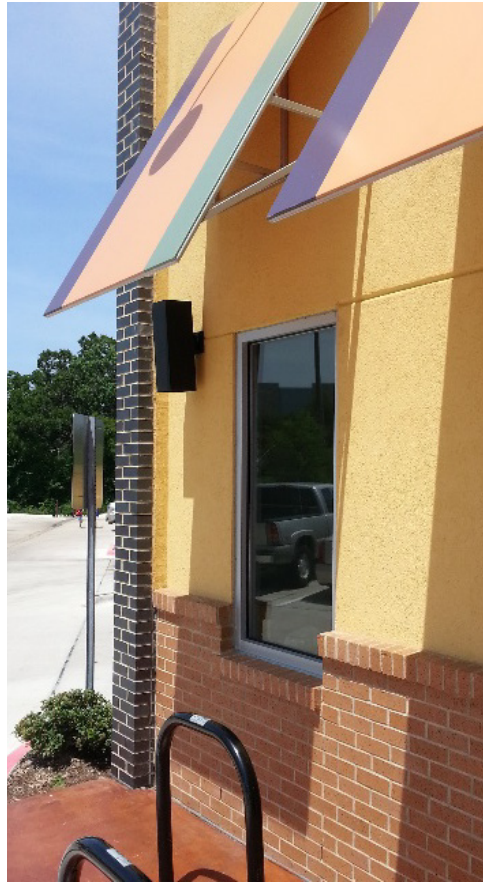
Fig. 9. Shadow Pattern Cast on an Exemplar IG Unit
