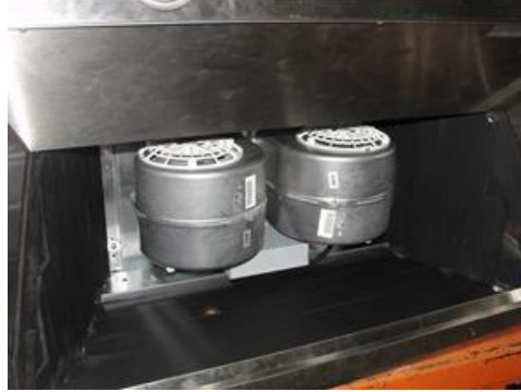
Figure 18: Range Hood Enclosure Modification (Code: ENC)
