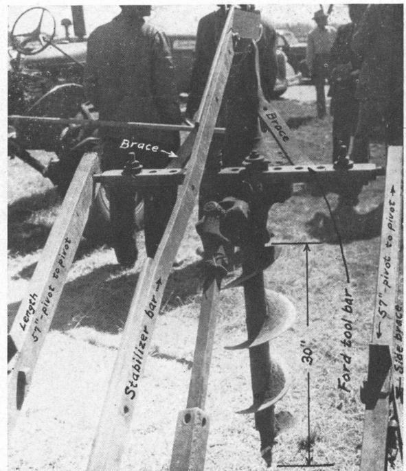
The rear end of a Model A Ford provides a basis for this digger. The top axle is cut off flush with the housing and welded to the housing to keep it from turning. A pipe to which a gin auger is welded is fitted over the remaining axle. Cutting blades are welded on at the tip to make the digger take the ground.
