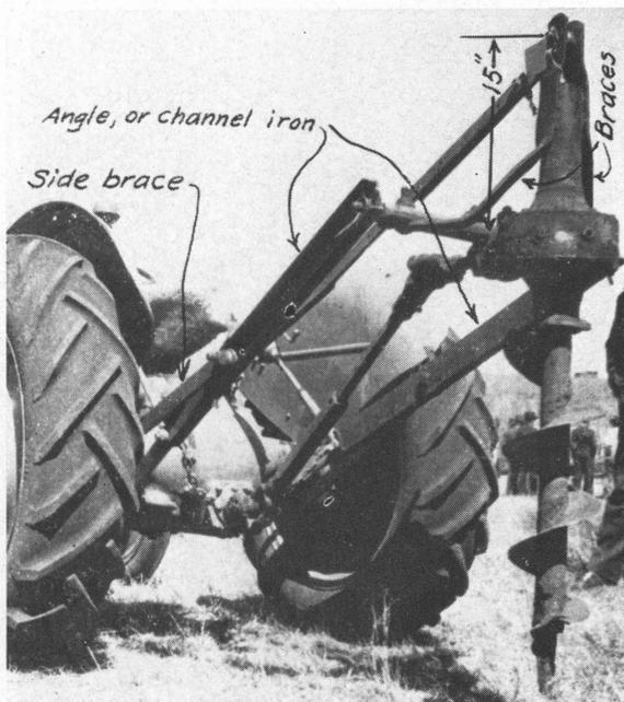
This post-hole digger was developed by Jack Woodson, foreman of the Circle Bar Ranch in Lubbock County. It digs holes 30 inches deep at the rate of two per minute. This machine was built entirely of scrapped materials. The only cost was for welding.
