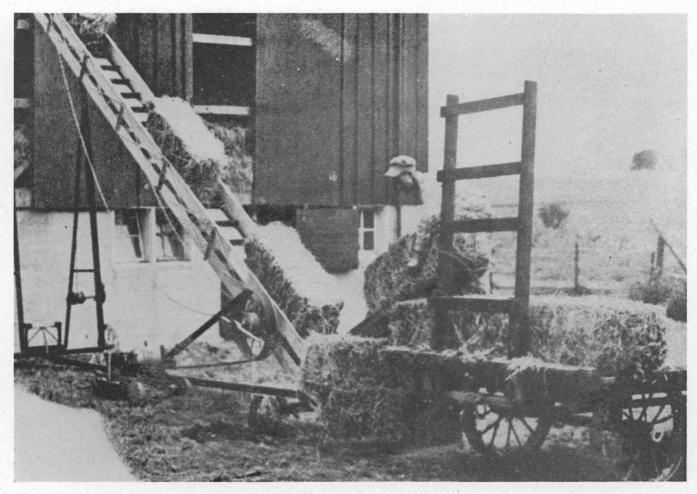
Portable bale elevator shown in operation. (Courtesy Public Service Co. of Northern Illinois)
