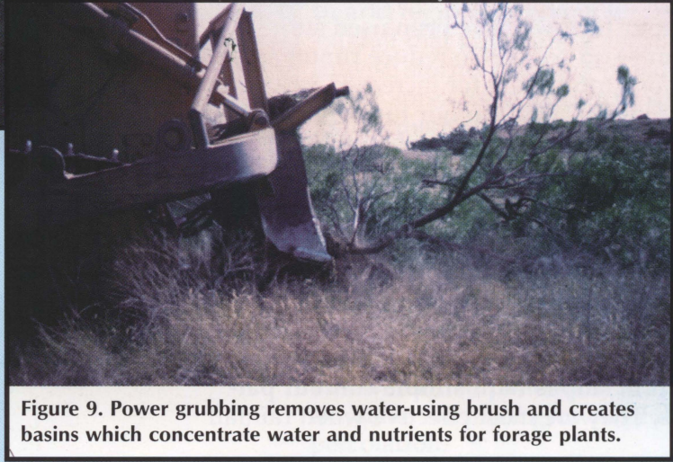
Figure 9. Power grubbing removes water-using brush and creates basins which concentrate water and nutrients for forage plants.
