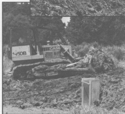
Depressional wetlands can be enhanced by shoveling levees closed (top), building up exterior levees with levee plows (middle) or installing water control structures (bottom).
