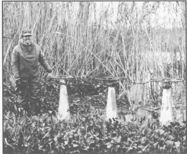
Water control structures such as flashboard risers (top), screw gates (middle) and concrete boxes (bottom) are used in wetland development projects.
