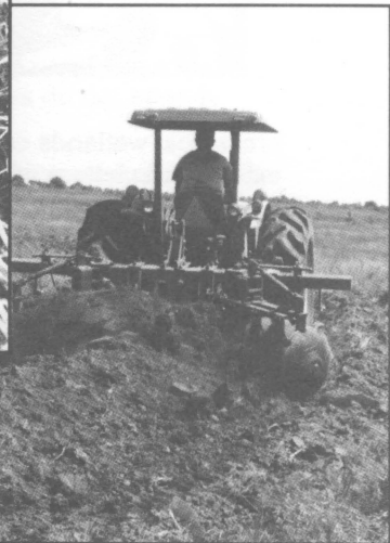
Depressional wetlands can be enhanced by shoveling levees closed (top), building up exterior levees with levee plows (middle) or installing water control structures (bottom).
