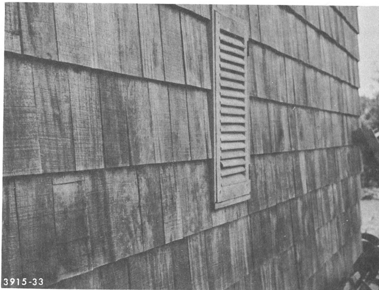
(c) Wood shingles for walls or roofs that have had trouble gaining general acceptability
