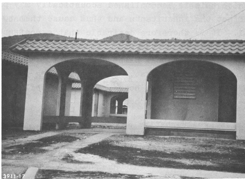
(b) Simulated tile roof of cast concrete
