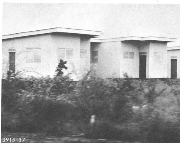
(c) More recent construction at TEMA where CGI and cement-asbestos roofing is used
