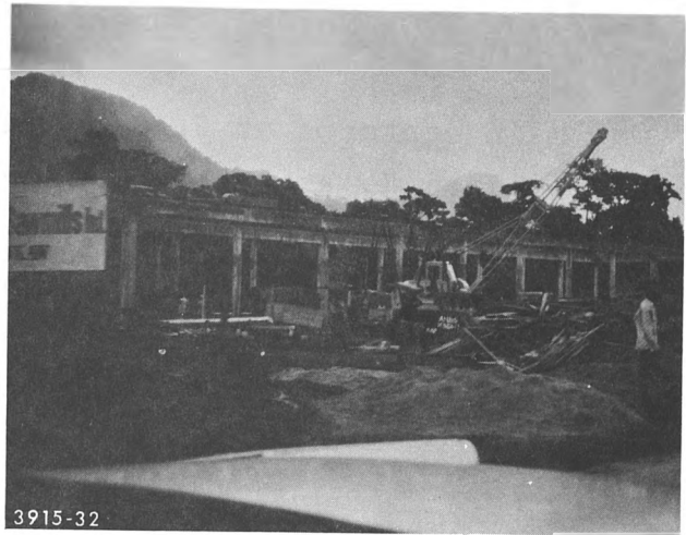
(b) Lumber mill showing sawdust residue
