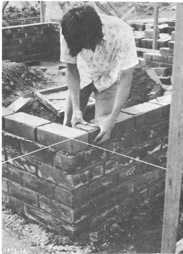
(a) Soil-cement (9/1 ratio) blocks being placed
