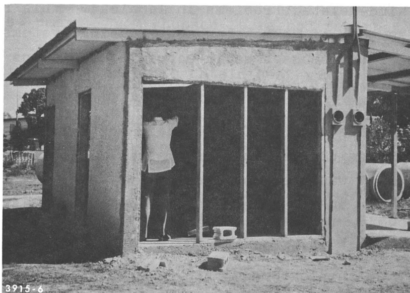
(b) Roughed in, steel-framed 200 square foot core
