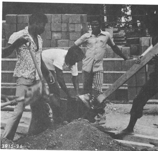
(b) Block press in operation to compress clay (UST)
