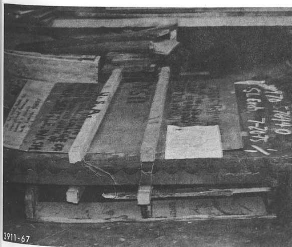
(b) Typical full scale (~50 in.) corrugated mold
