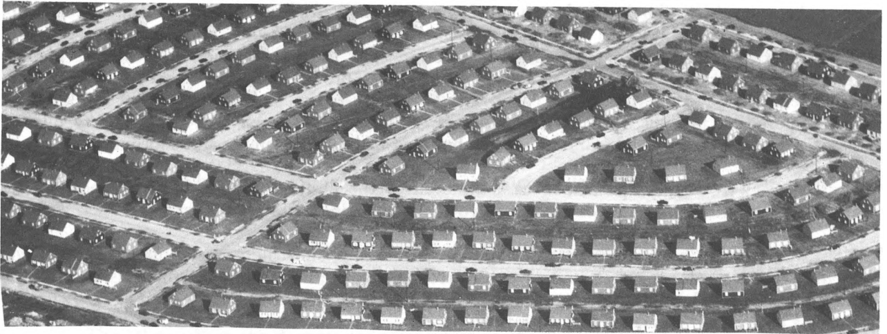
MASS-PRODUCED, CONVENTIONAL DWELLINGS – These U.S. tract-houses epitomize the industrialization of process, while holding product technology at conventional levels. These standardized, traditional houses were mass-produced at Levittown, Long Island, in 1947, utilizing highly-specialized and coordinated labor teams which moved from house to house at virtually an assembly line pace. (Levitt and Sons photo)
