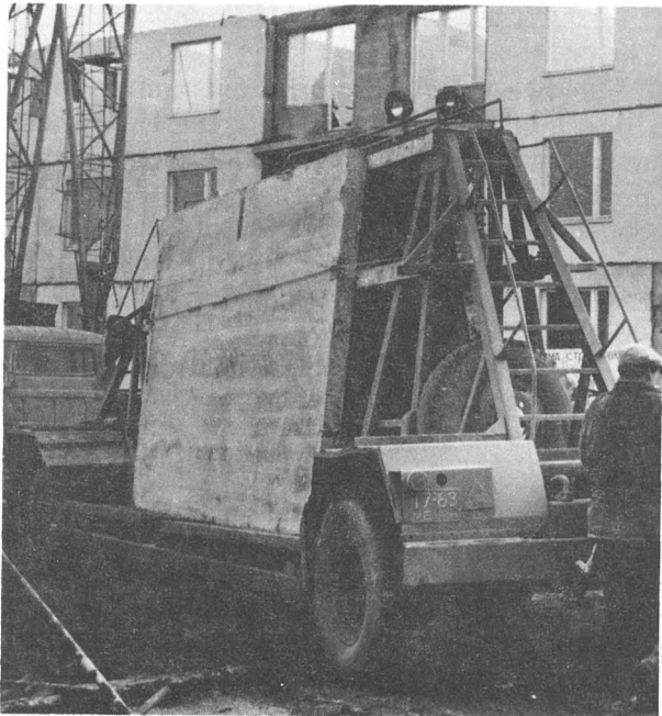
SOVIET INDUSTRIALIZED HOUSING — Completed bath units are loaded from storage onto trucks (above), while wall panels arrive on site (below left) and are then lifted into place by crane (below right).
