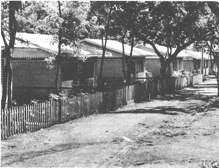
View of typical house at Colonia Managua, Nicaragua (1959)
