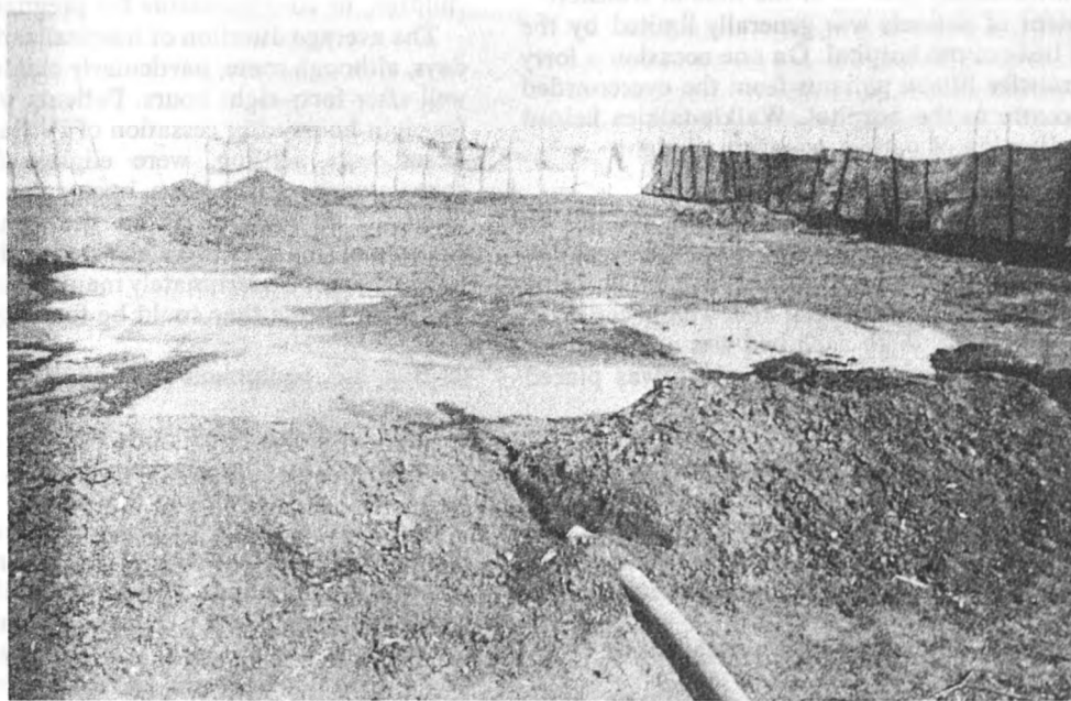
Fig. 4. Evaporation lake for disposal of chlorinated waste washing water.
