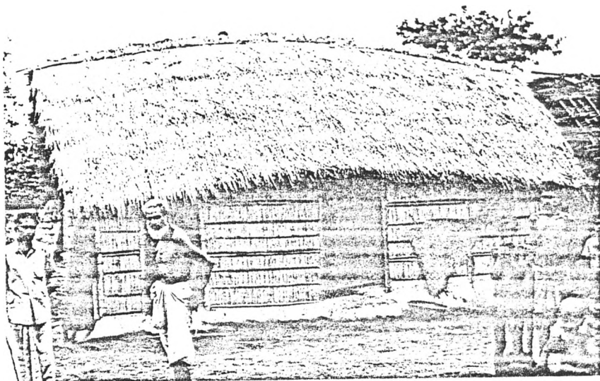
Indigenous Village Housing in Khunda in Bramanbaria Area 18. Well-maintained house
