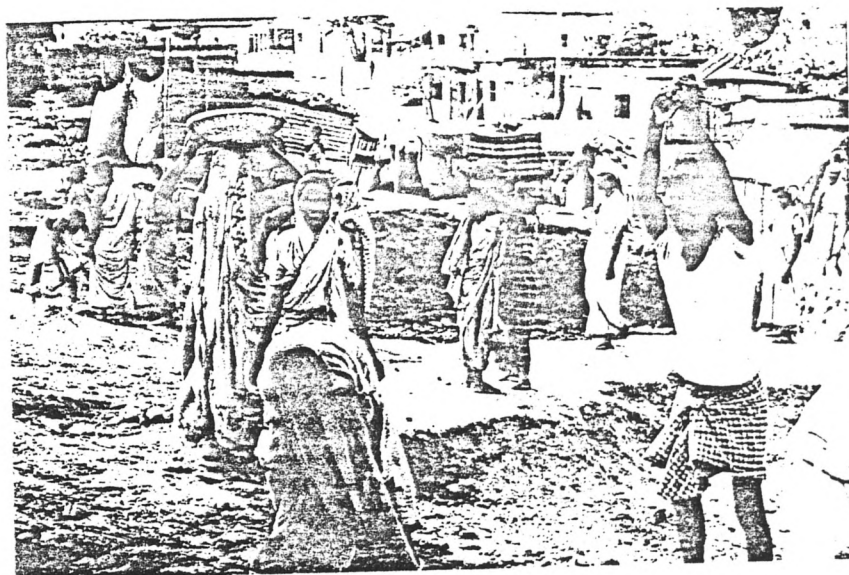
2. Work in progress- Levelling of land
