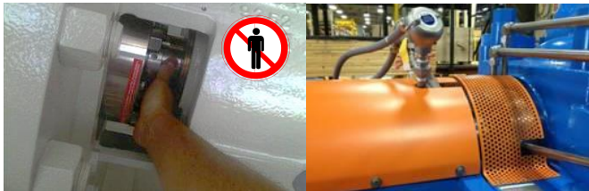
Figure 1: Unguarded shaft area vs. guarded
