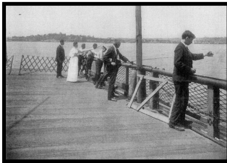
Figure 12. Transverse decking on the outside deck of Southfield II (Allen 1909:202).
