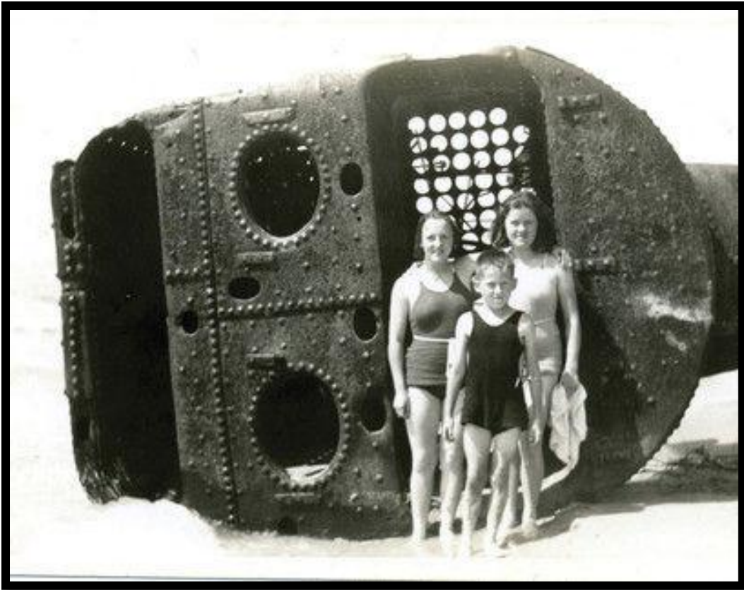
Figure 135. Tipped over boiler with separate fire door and ash pit frames (Image of boiler from Erie Belle shipwreck, located in Lake Huron; courtesy of Kathryn Houston and the Walker House Hotel in Kincardine, Ontario).
