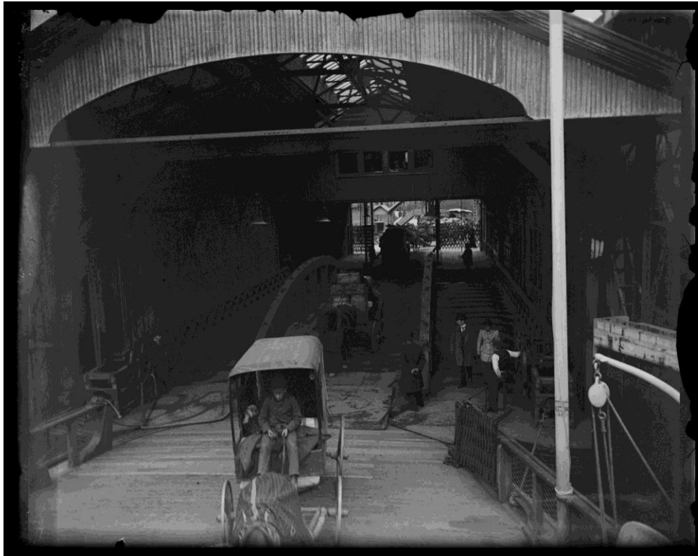
Figure 6. Unidentified Staten Island ferry docked in berth that matched the shape of the double-ended bow and stern (Image courtesy of Historic Richmond Town, Staten Island, NY.; reference # 50.15.6033).
