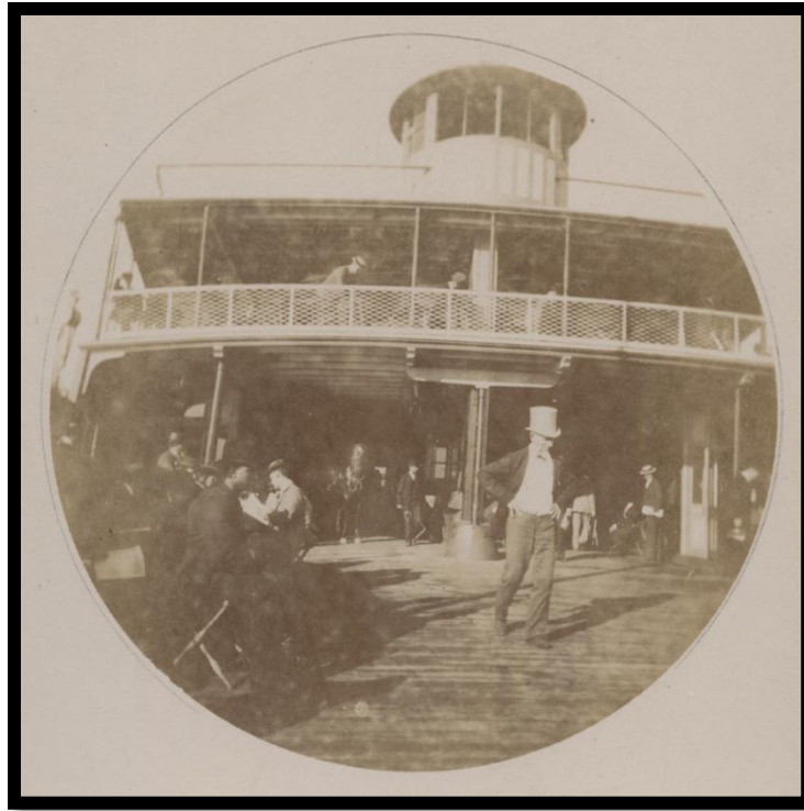
Figure 11. Transverse decking on the outside deck of Northfield (Image courtesy of Historic Richmond Town, Staten Island, NY.; not yet cataloged, reference: Ferry Northfield , Tompkinsville Landing [man wearing top hat], August 16, 1892).
