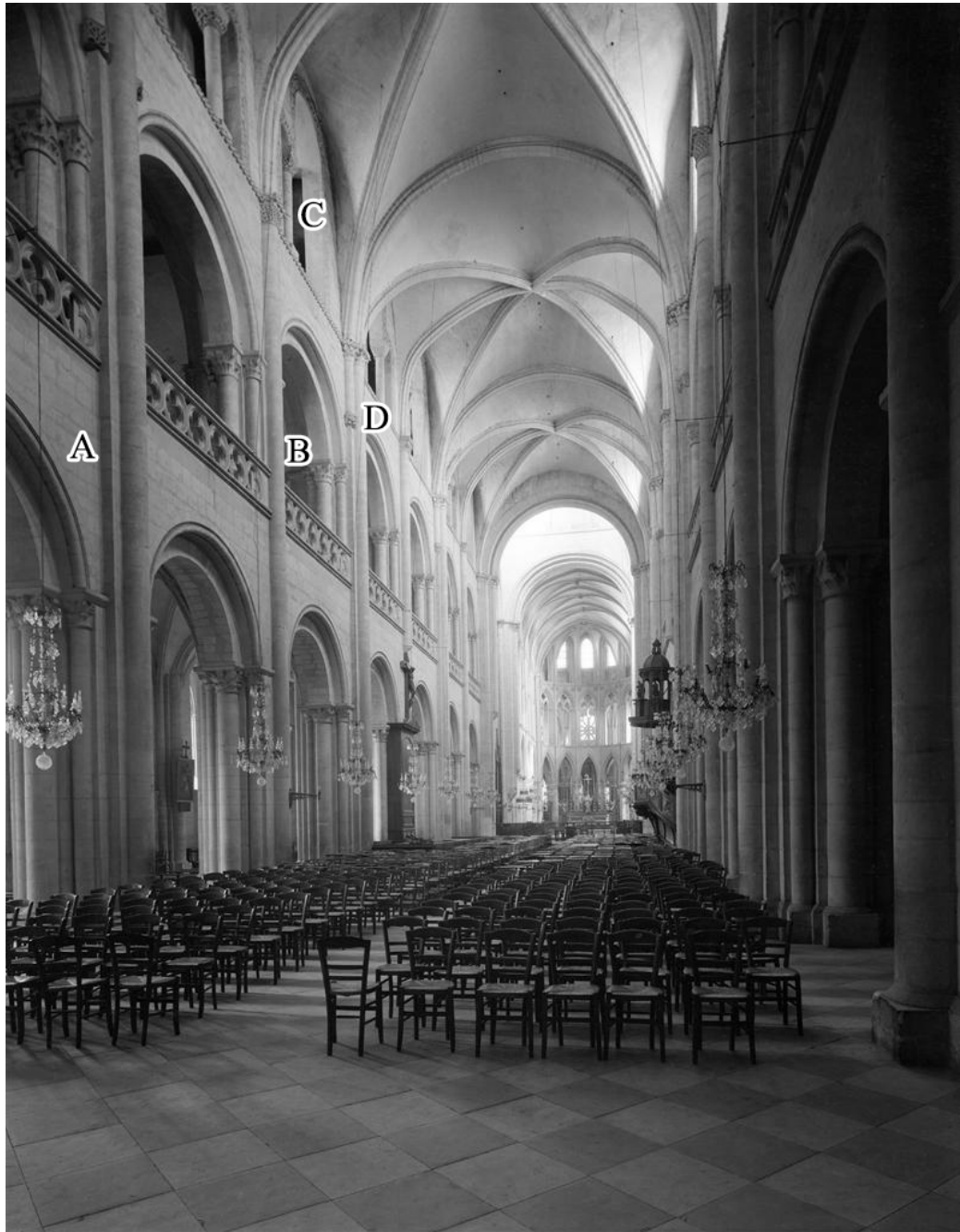
Figure 4.11 St. Étienne Nave Interior (copyright National Gallery of Art, Washington DC). A=piers; B=gallery; C=clerestory; D=clustered columns supporting ribs.
