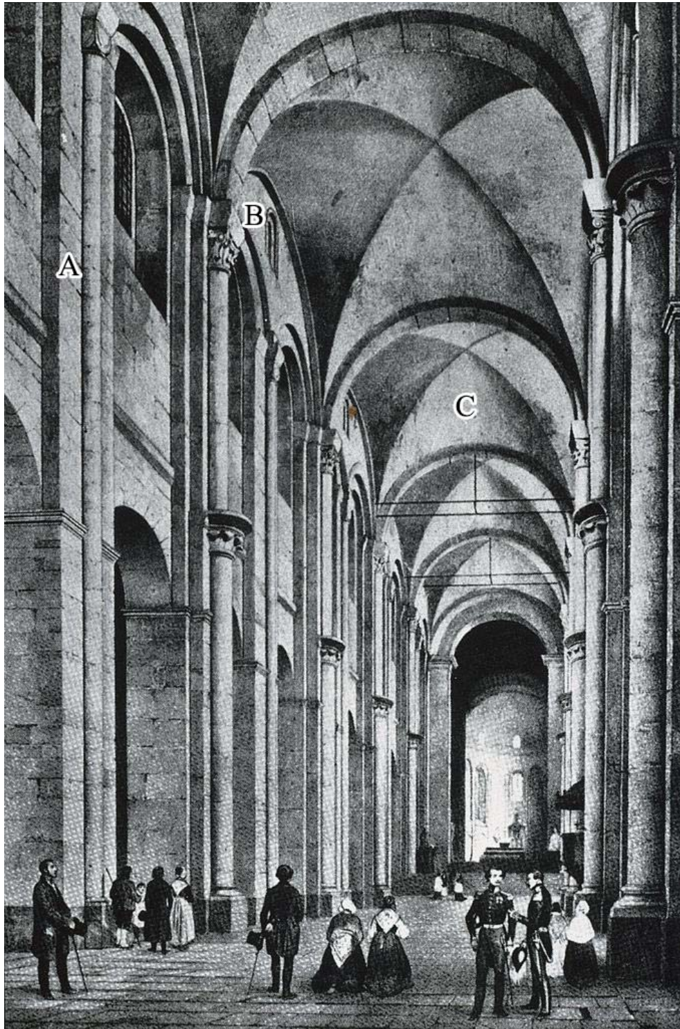
Figure 4.8 Interior of Speyer Cathedral, before 19 th century renovations (copyright University of California, San Diego). A=large piers with half columns; B=arches above clerestory; C=groin vaults.
