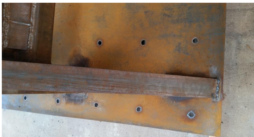
Figure 85. Series of \frac{3}{4} " holes torched into the \frac{1}{2} " thick base plate of a secondary stand.
