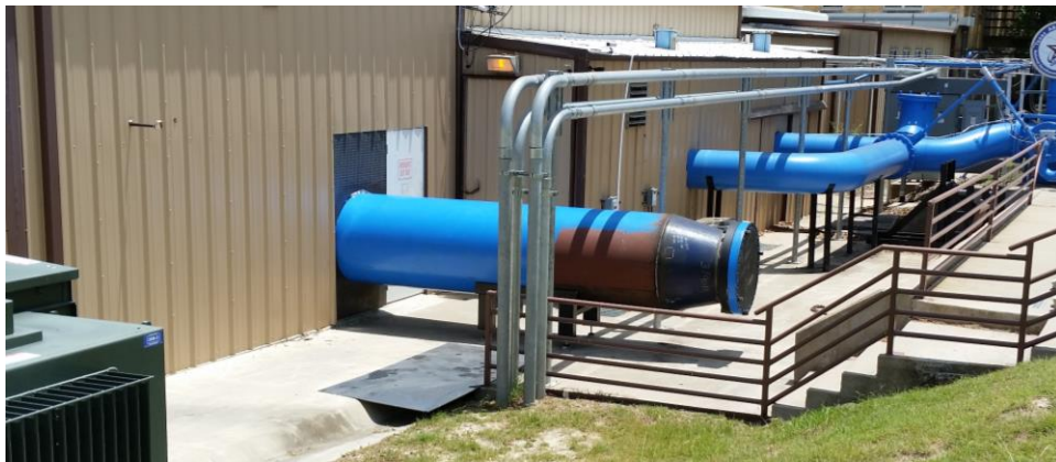
Figure 62. Tailpipe as it was installed through the wall at the NAL.
