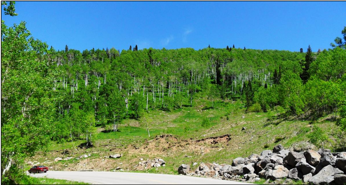
Figure 6. CDOT management of the DDLC. Debris is removed from the road and stockpiled (6a) while concrete barriers and boulder rip-rap are used to stabilize the toe. July 2011.
