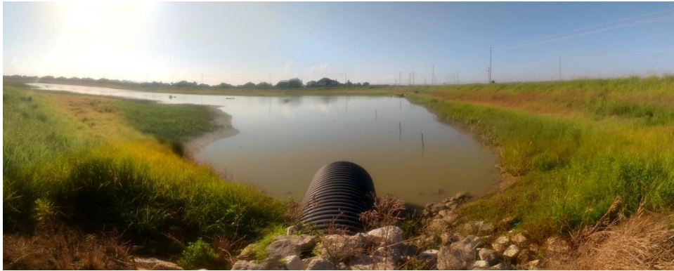
Figure 11 – The view from this inlet shows an inlet and the littoral zone that floods after a storm event.
