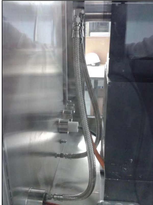
Figure 3-22: The inlet and outlet water lines connecting to the motorized spindle through the bulkhead
