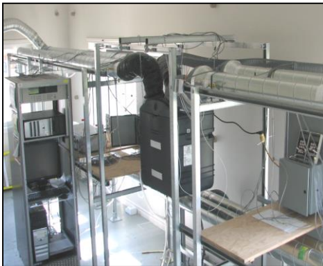
HRV/ERV Test Rig
