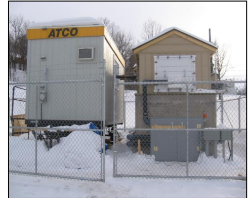
Radon Test Facility
