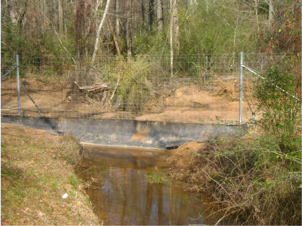
Attoyac Bayou at US 84 (20842), 2/8/2012 addition of silt screen and game fence.
