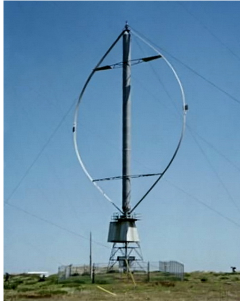
Figure 1.5: Darrieus Turbine
