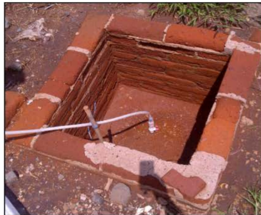
D. Jarrero well chlorination system part b.
