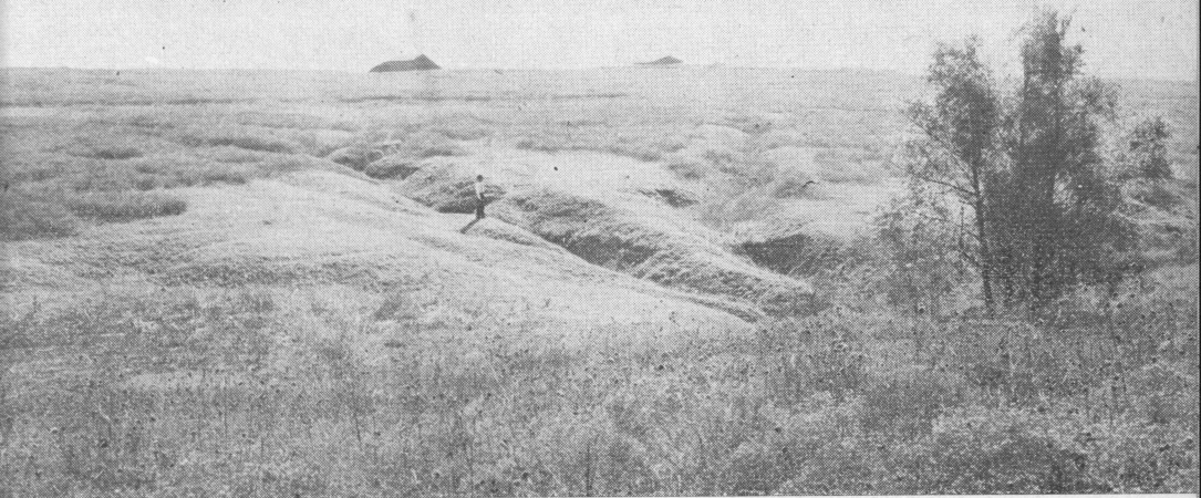
Fig. 10. Gullies shown in Fig. 9 have been brought under control. The steep banks of the gully channels are protected by Bermuda grass. The area surrounding the deep cuts is covered with a good stand of buffalo grass. Sodding and good pasture management have halted erosion. Mowing is needed in the remainder of the pasture to control weeds.
