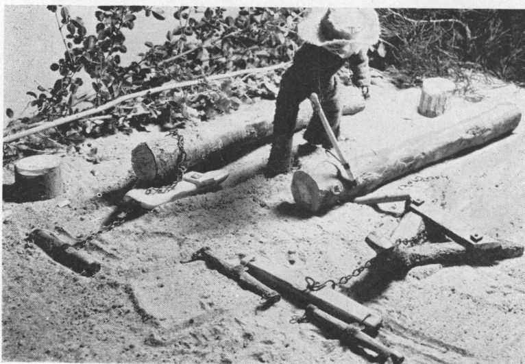
Fig. 14. Skidding lizards are loaded by roll-up or by a method used with bumpers. The choke hook end of pulling chain grips the log to the bunk.
