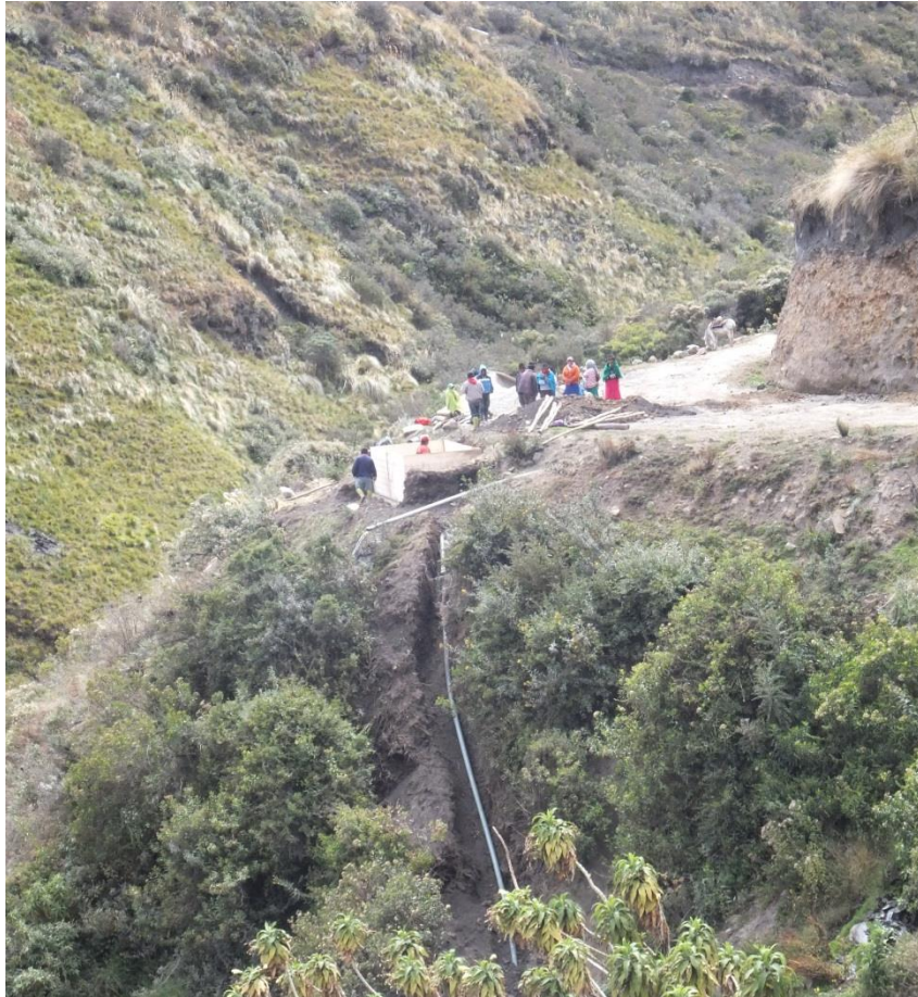
Figure 5.7 Minga to construct the water holding tank in Quinchucajas (September 2013)
