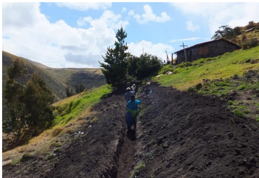
Figure 5.6 Digging the irrigation canal in Quinchucajas (August 2013)
