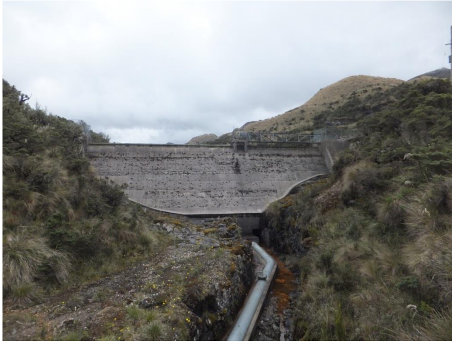
Figure 3.3 The Loreta Reservoir dam in the páramo, Cayambe-Coca National Park (November 2012)
