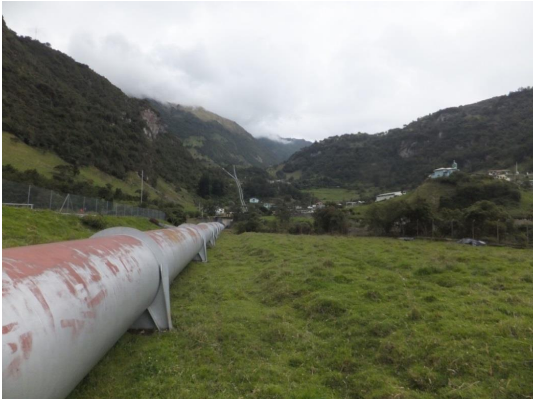
Figure 3.2 Water pipeline to Quito passing through the town of Papallacta (November 2012)
