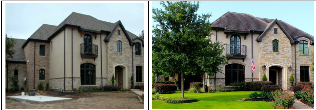
Figure 34. Pre-landscape with water collection cistern installed (left image) and landscape fully mature (right image)
