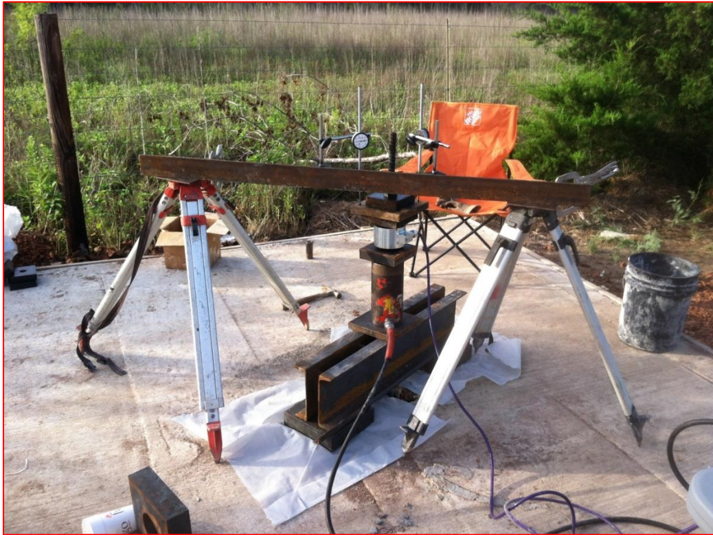
Figure 7-24. Soil nail pullout test setup
