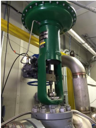
Figure 21. Control valve on outlet line
