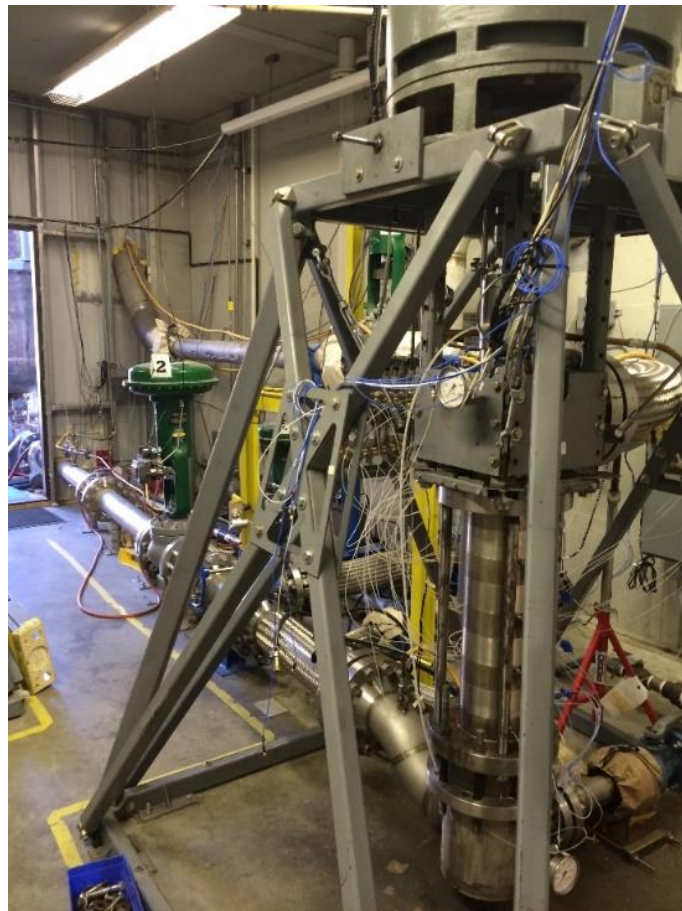
Figure 25. Inside of closed loop test facility. Pump is beneath motor stand (right). Control valves and inlet/exit piping are at left.
