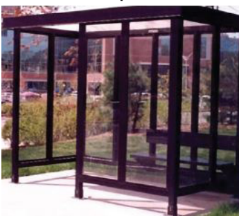
FIGURE 4.33: Example of Bus Shelter
