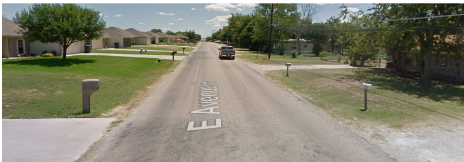
FIGURE 4.8: East Avenue H
