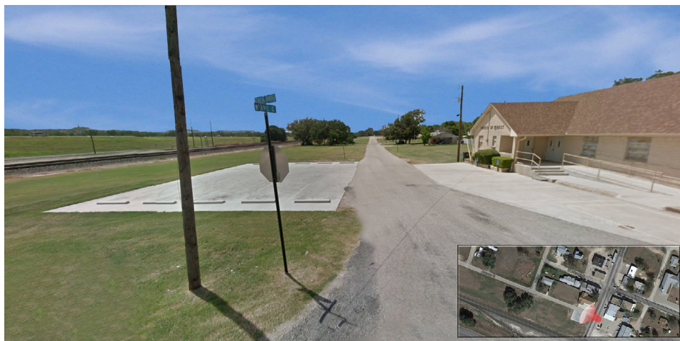
FIGURE 4.10: Avenue G Before (top) and After (bottom)
