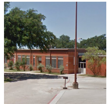
FIGURE 1.1: Nolanville's new city hall
