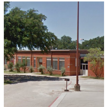
FIGURE 1.1: Nolanville's new city hall
