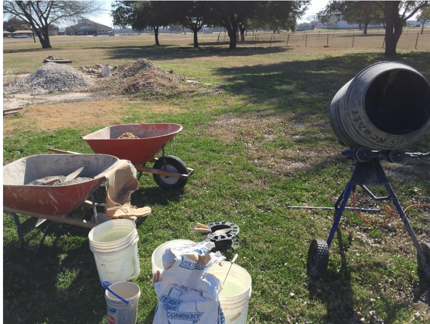
Figure 19: Concrete mixer, cement and sand
