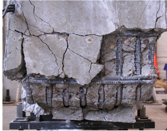
(b) Specimen 2: Slight ASR/DEF Damage
