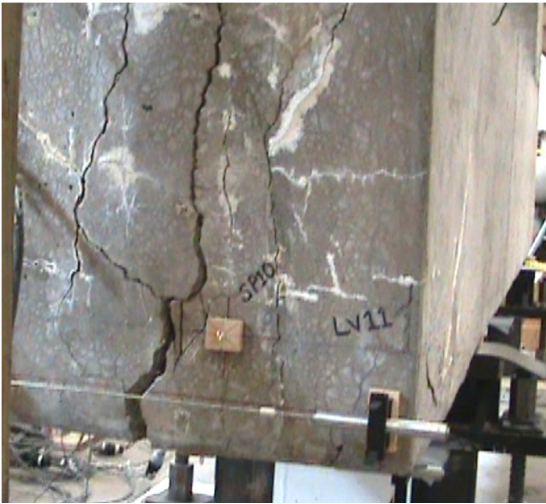
(c) At 2215 kN (Just before Failure)
