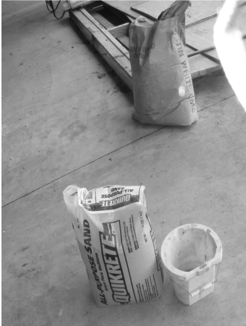
Figure 22: Sand and lime
