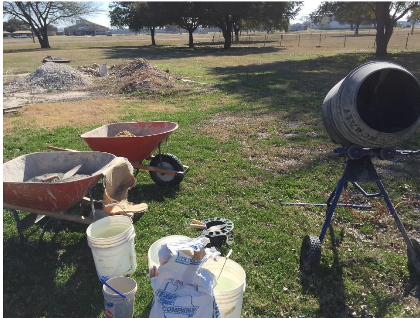
Figure 19: Concrete mixer, cement and sand
