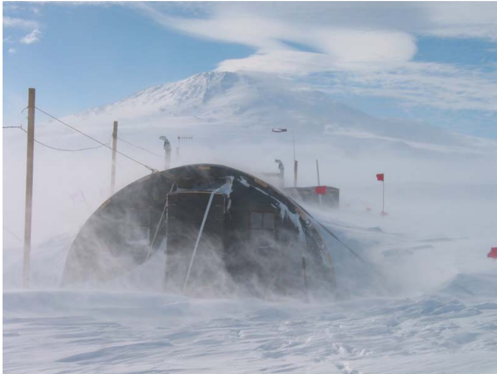
Figure A- 69: Wind batters a Jamesway structure in a field camp outside McMurdo Station (Mt Erebus in the background) in 2001.
