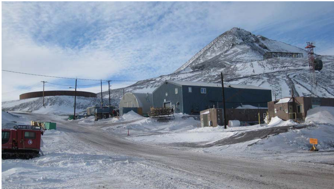
Figure A- 54: Observation Hill, on the southwest side of the station. Photo by author, 2010.
