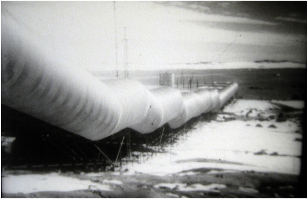
Figure A- 40: Casey Station, Antarctica. A view of the tubular shield and buildings on silts, which protect the buildings from an accumulation of snow on the Australian base. 2-27-74. Photo by PH2 Michael C. Wright, Official U.S. Navy Photograph. Courtesy U.S. national Archives, College Park, MD.
