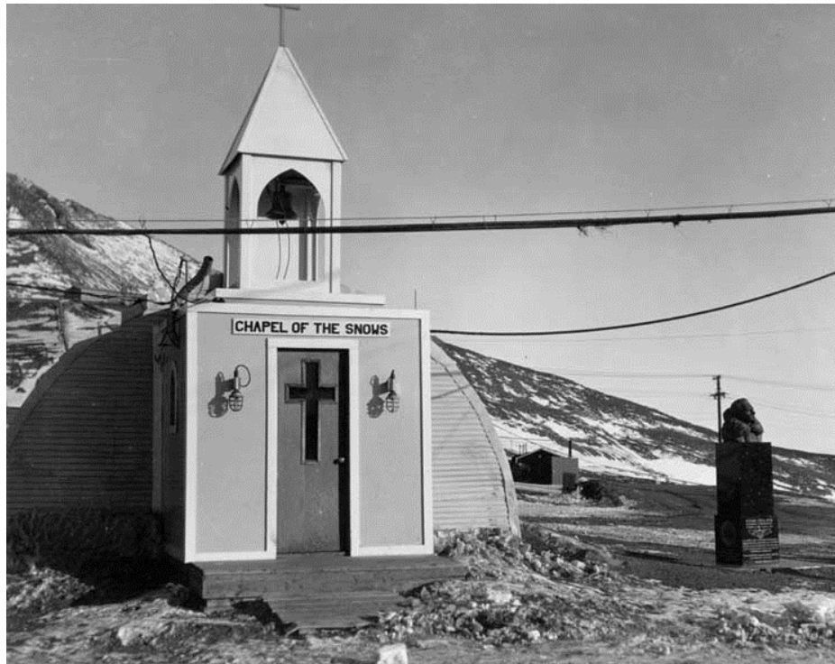
Figure A- 2: The original "Chapel of the Snows" at McMurdo Station, Antarctica, 1965. Quonset hut with vestibule entrance. Official U.S. Navy photograph, National Archives collection.
