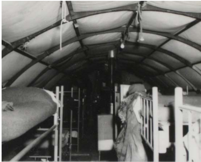
Figure A- 22: Cargo handler battalion One CHB-1 Barrack. Floor space is 16 ft. x 52 ft. with twenty bunks. McMurdo Station, Operation Deep Freeze '64. Photographer: PH2 D.C. Armstrong. Courtesy U.S. National Archives, College Park, MD. Accessed March, 2012.
