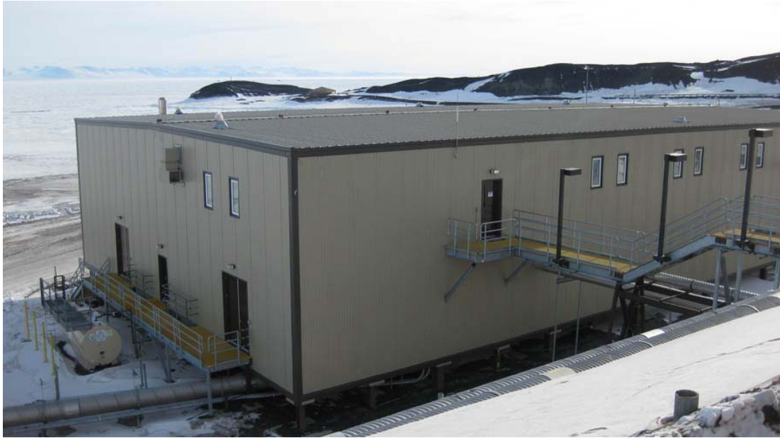
Figure A- 74: McMurdo Waste Water Treatment Facility, which sits at the edge of the coastline.
