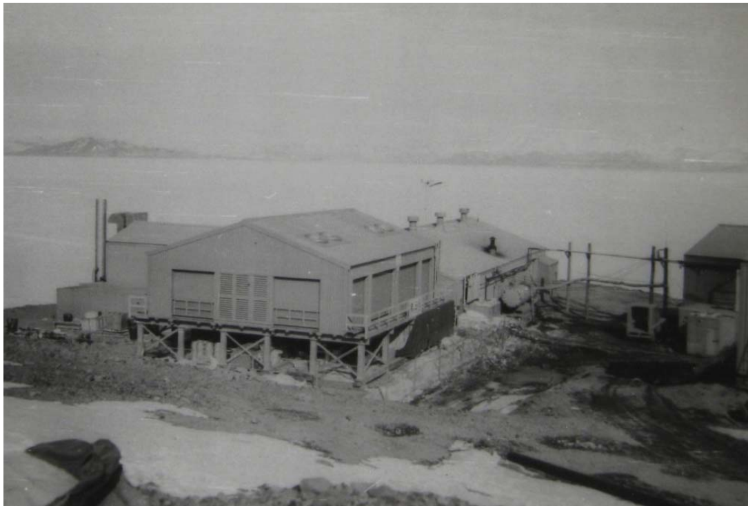
Figure A- 66: Power Plant—Nuclear PM-3A. McMurdo Station, Antarctica. Operation Deep Freeze '65.
