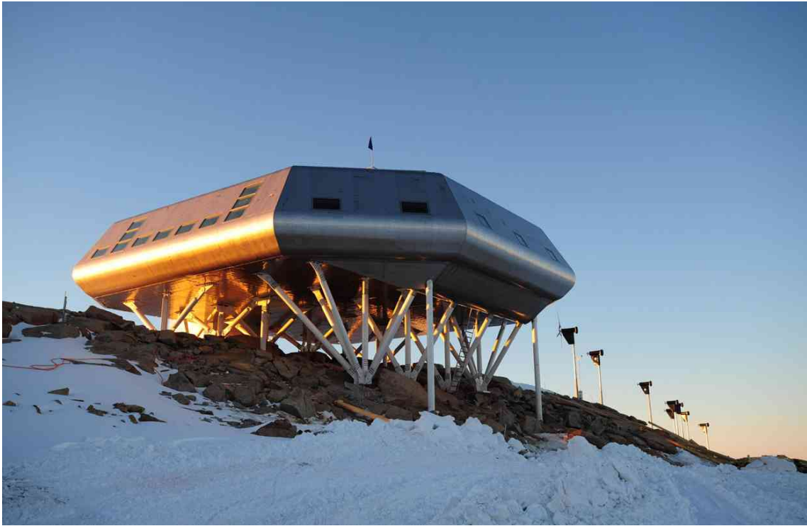
Figure A- 42: View of Princess Elisabeth station. Project © International Polar Foundation. Engineering and Technical Design for the Structure and the Shell © Philippe SAMYN and PARTNERS.
