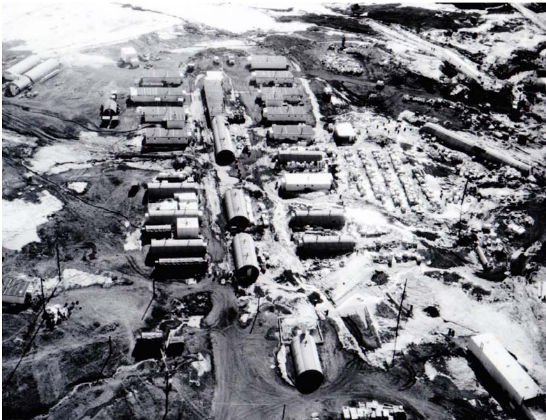
Figure A- 7: "Sky View McMurdo Sound Naval Air Facility." 1957.
