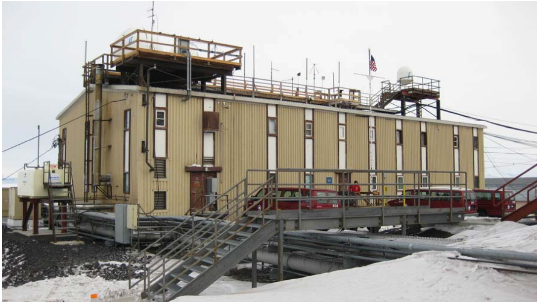
Figure A- 53: Pipes and a pedestrian bridge in front of Building 165, Mac Ops (Communications Building). Photo by author, September, 2009.
