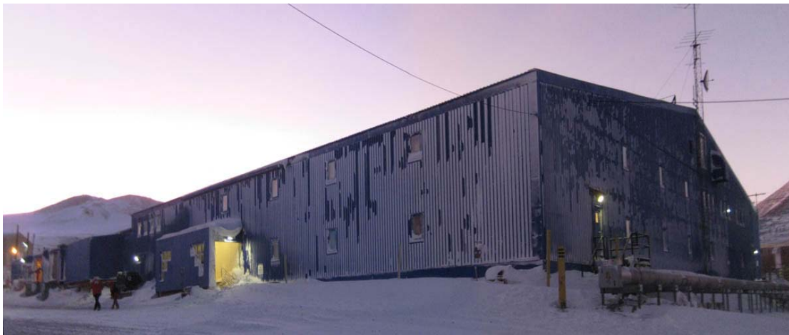
Figure A- 12: Building 155, now painted blue, after a wind event, August 2010. East side with entrance (left) and south side (right). Photo by author, 2010.
