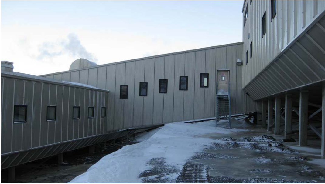
Figure A- 56: A long hallway with juxtaposed stairs and a ramp connects all three phases of the Crary lab as they descend the terrain of the coastline. Photo by author, 2010.
