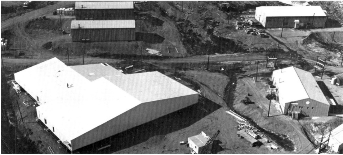
Figure A- 11: Building 155 halfway built, c. 1967. Pope, 1967, p. 139
