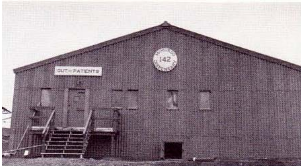
Figure A- 29: The Medical dispensary around 1968. This is one example of a Robertson building. The front door has changed some, but this building has stood since 1961. USN, 1968, p. 36.
