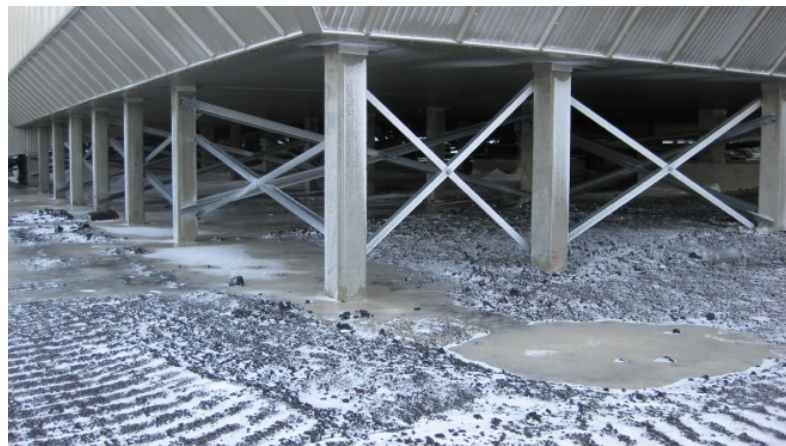
Figure A- 59: Example of a concrete footing in McMurdo Station. Photo by author, 2009.
