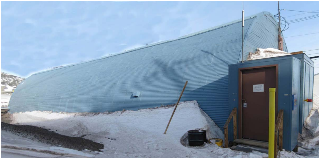
Figure A- 20: A Quonset hut in McMurdo Station with a vestibule entrance addition. Photo by author, 2009.
