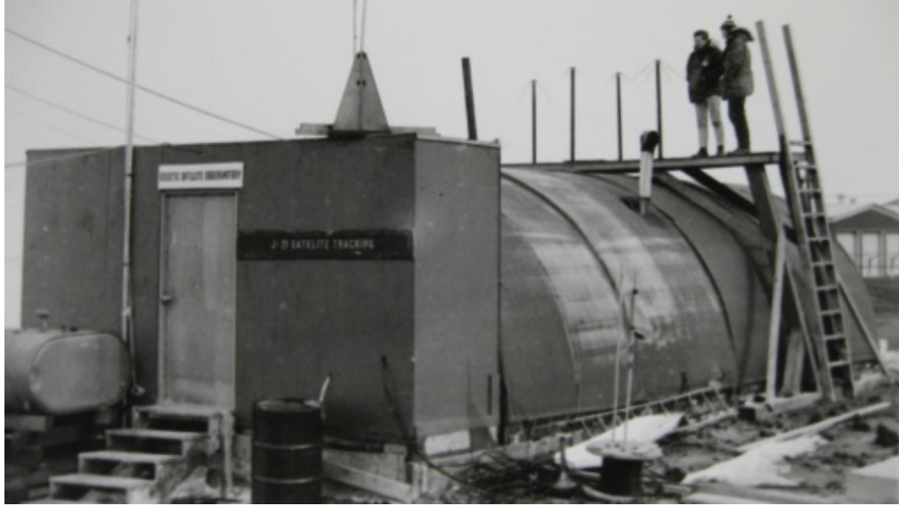
Figure A- 3: Two men stand on top of the Geodetic Satellite Tracking Building, McMurdo Station Antarctica, 1973. Courtesy U.S. National Archives, College Park, MD. Accessed March, 2012.
