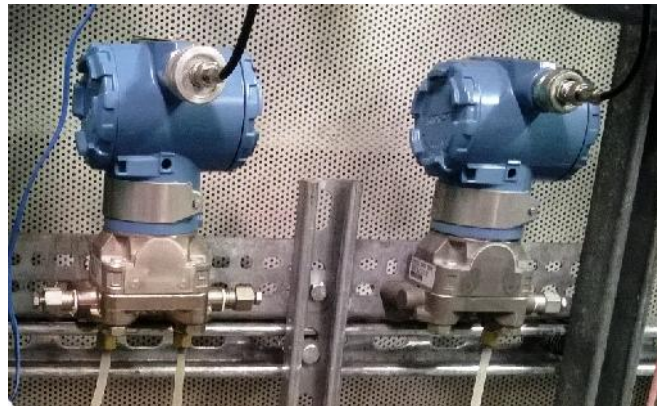
Figure 4.7 Pressure and DP Transducer
