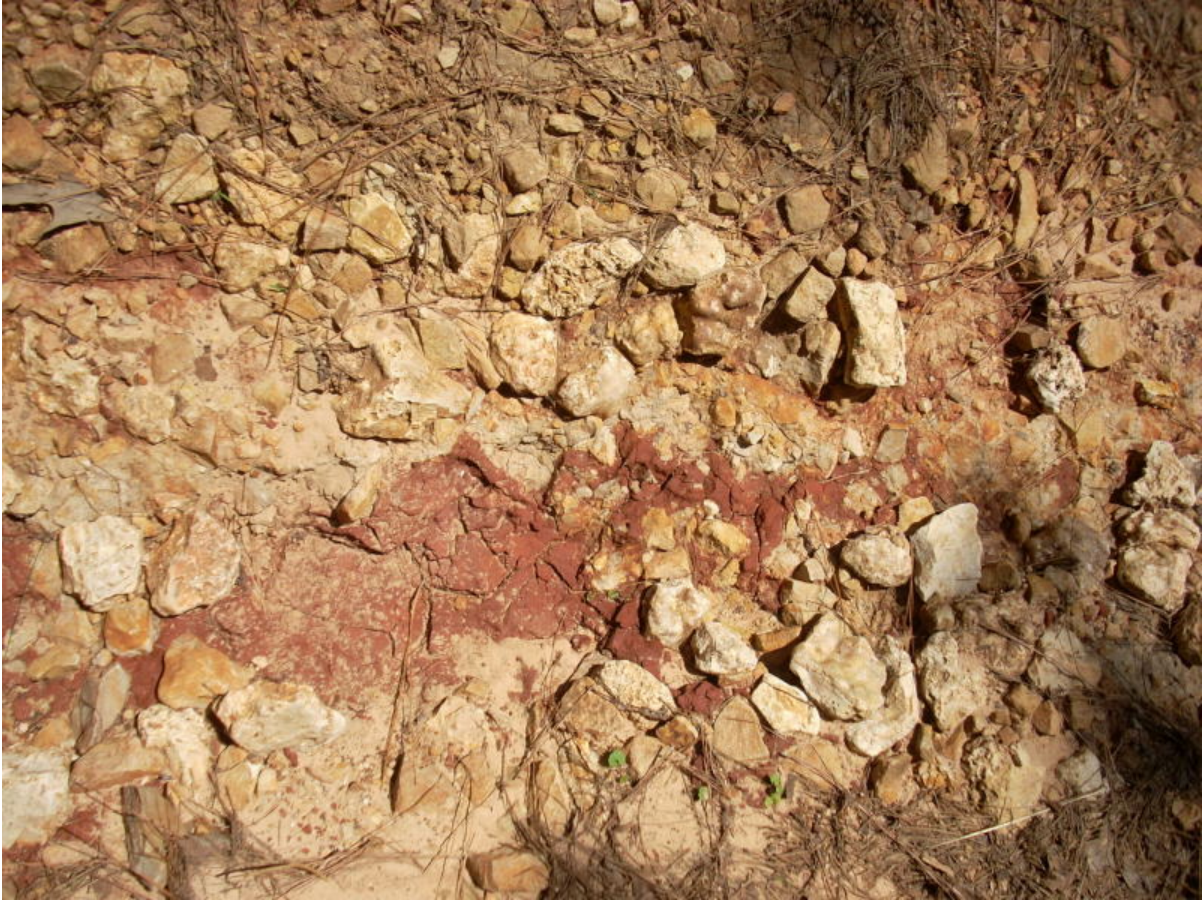
Figure 6. View of Clay at Surface of Road (mixed with gravels)
