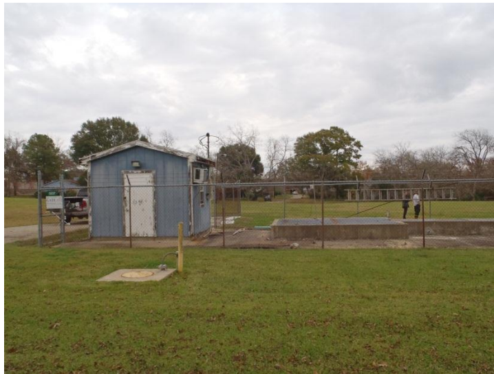
Figure 5 - Municipal water building near Chappell Hill St.
