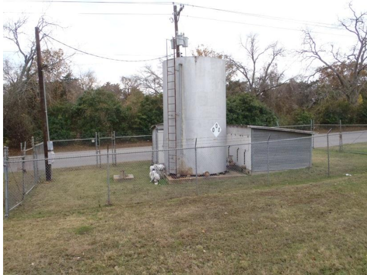
Figure 4 - Municipal water building near Chappell Hill St.
