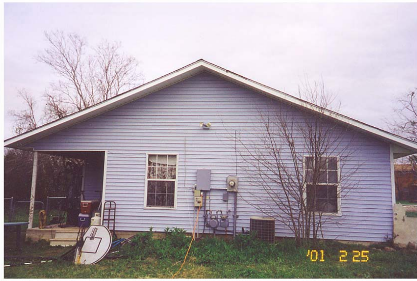
Figure 3.6 – Photograph of the back elevation of the case study house (facing southwest).
