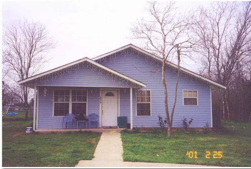
Figure 3.5 – Photograph of the front elevation of the case study house (facing northeast). The photograph was taken on February 25 th , 2001 at the case study site.
