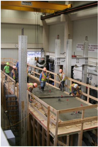
(b) Finishing the deck
