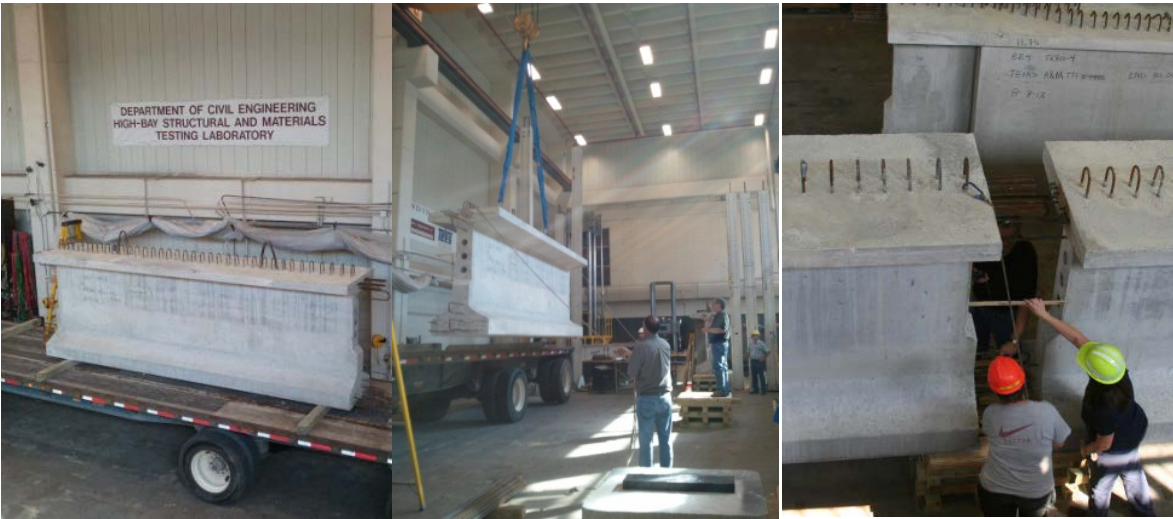
(a) Girder segments with lifting points
