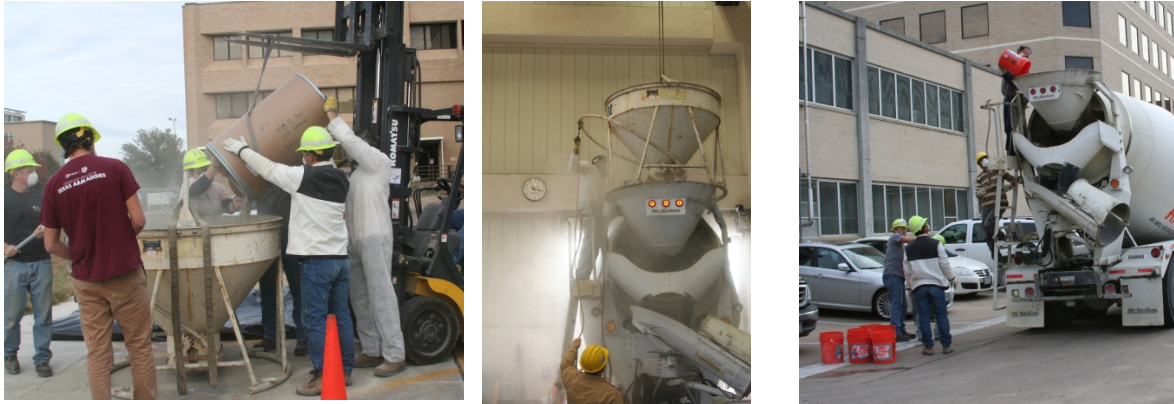
(a) Measuring cement into hopper
