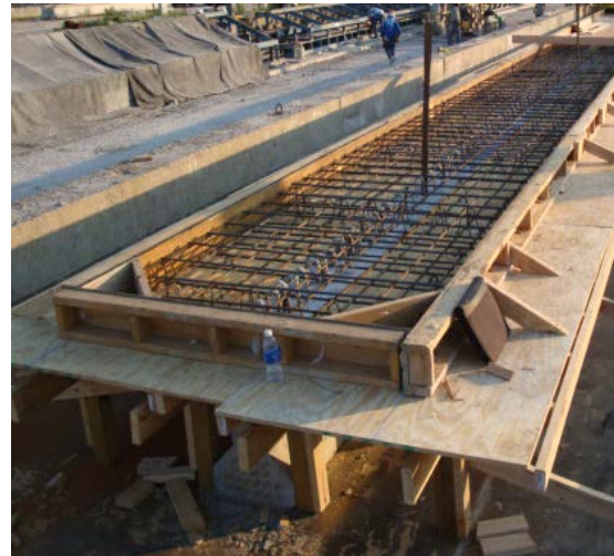
(b) Deck mild steel reinforcement
