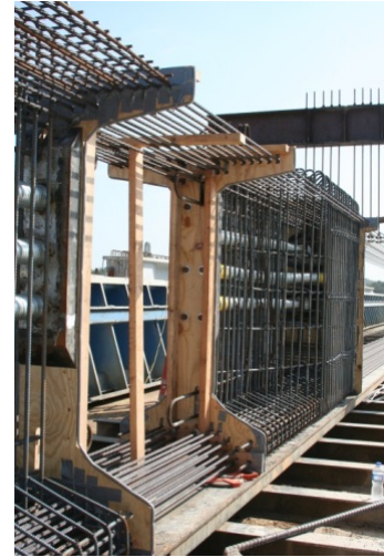
(b) End block reinforcement
