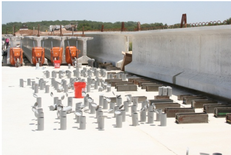
Figure 5.2. Preparation for Fabrication of Girder Test Samples.
