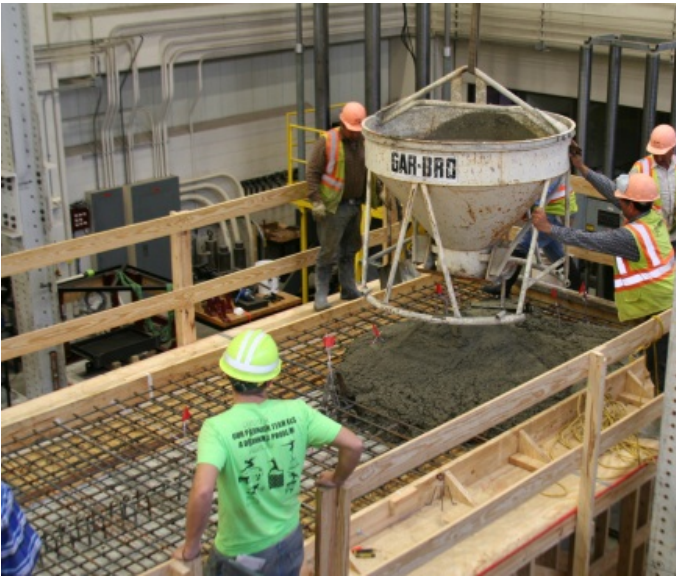
(a) Casting the deck
