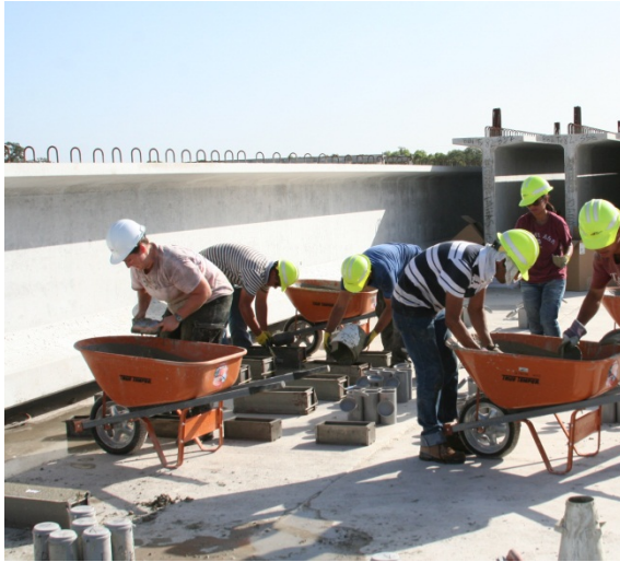
(a) Sample of batch concrete fills 3 to 4 wheelbarrows
