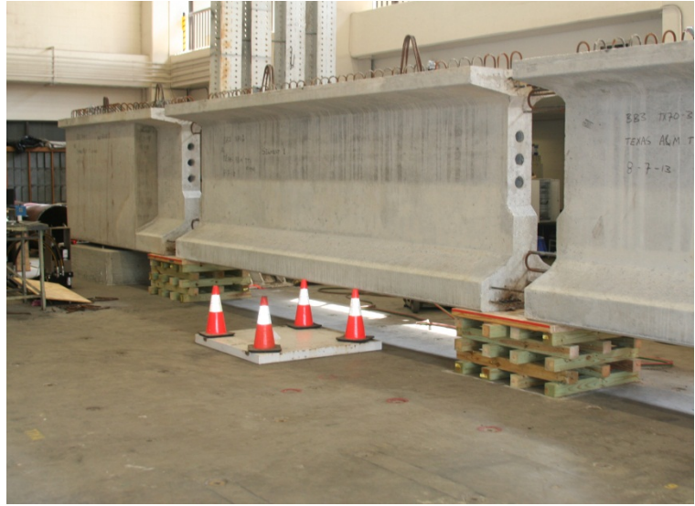
(b) Side view girder alignment
