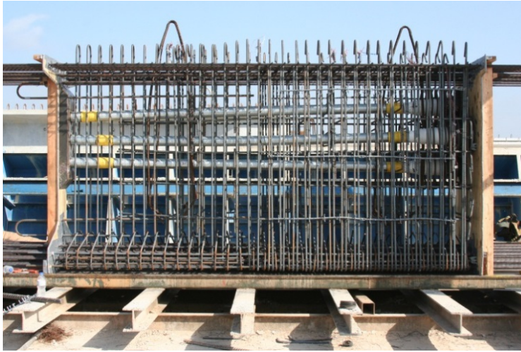
(a) Interior segment reinforcement
