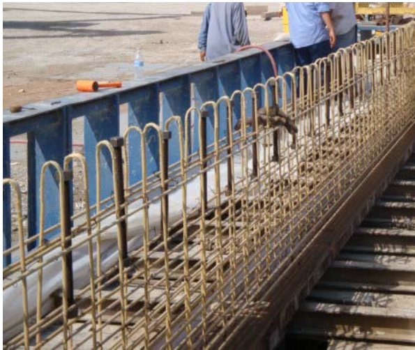
(a) Girder AFRP reinforcement
