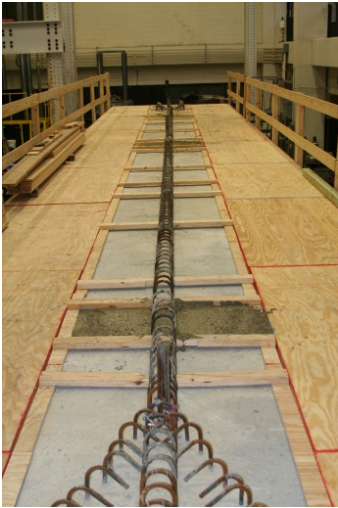
(b) Casting connections complete
