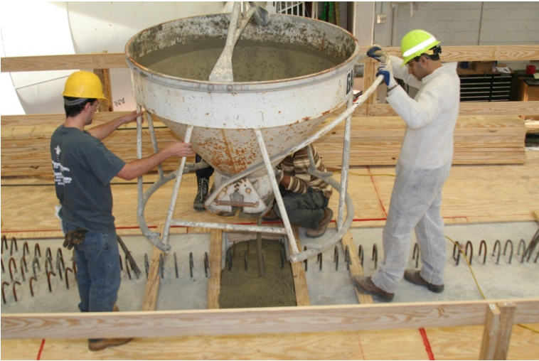
(a) Casting connection
