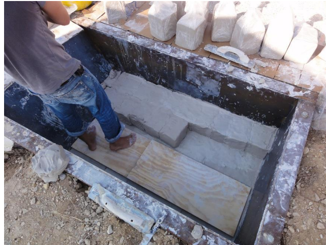
Figure 3-26: Soft clay placing inside the trench box
