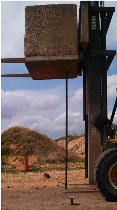
Figure 3-31: Boring preparation for PMT in hard clay
