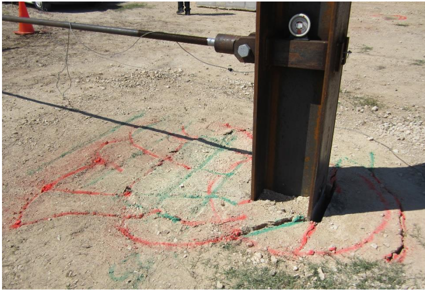
Figure 3-69: Soil deformation in static test for pile in very dense crushed limestone
