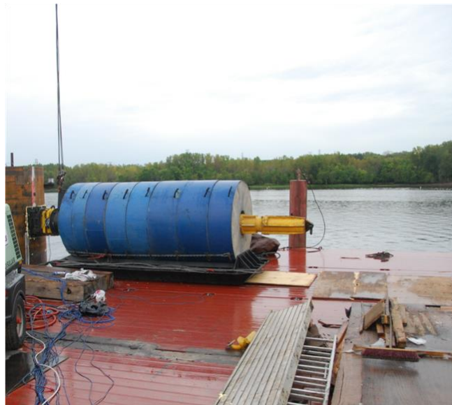
Figure 2-2: Lateral Statnamic loading test (Applied Foundation Testing 2012).
