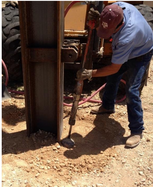
Figure 3-34: Soil compaction during the post installation using a mechanical tamper
