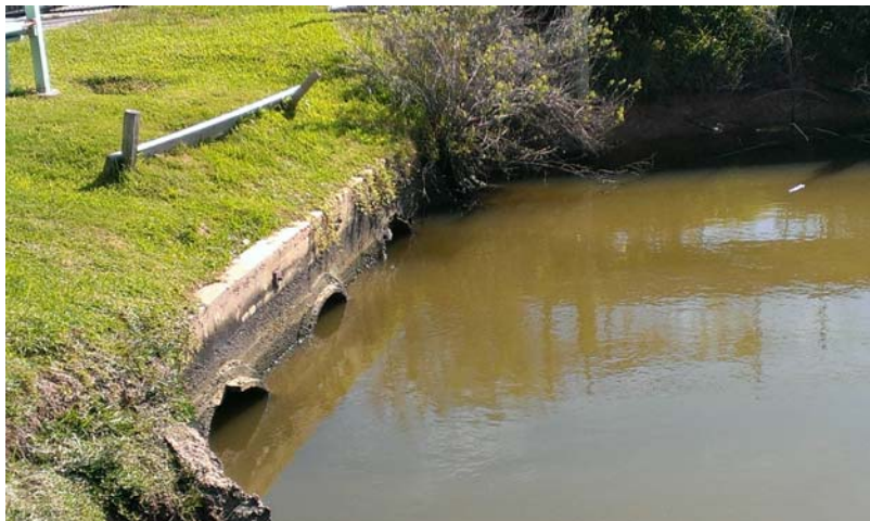
Figure 3.2. Stormwater retention pond side, culverts connecting marina and stormwater retention pond.
