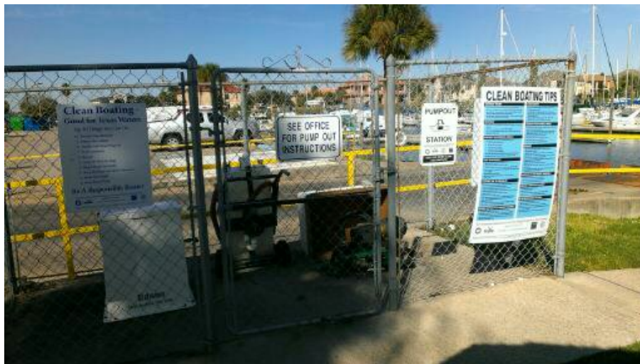
Figure 2.1. Pump-out station and mobile pump-out cart at Marina Del Sol.
