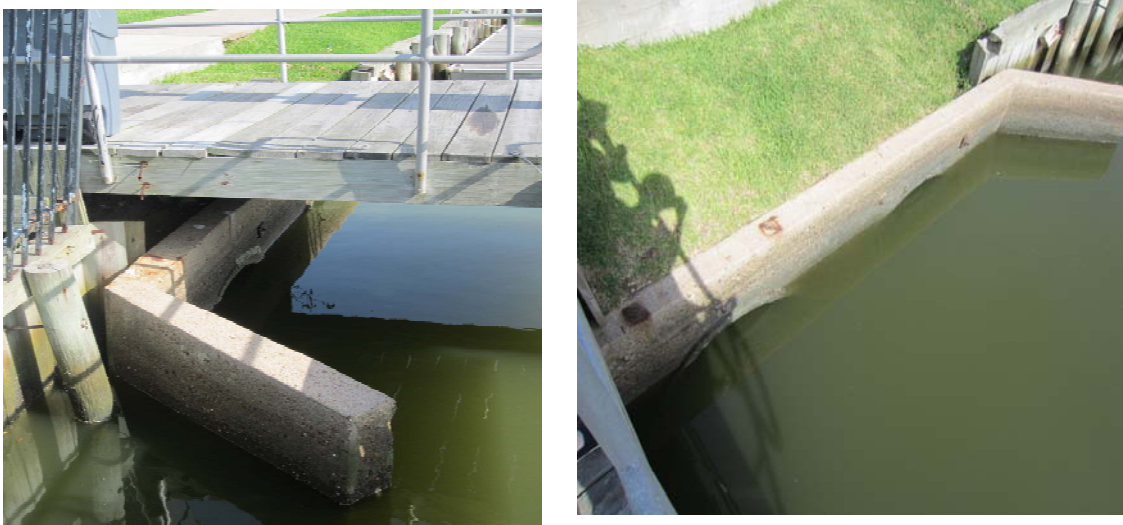
Figure 2.19. Marina side, culverts connecting marina and stormwater retention pond.
