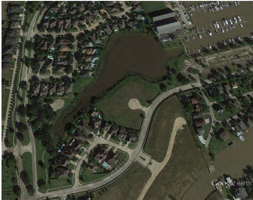
Figure 3.1. Stormwater retention pond located west of Marina Del Sol.
