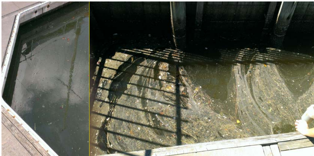
Figure 2.4. Organic debris collecting in poorly circulated areas of Marina Del Sol.
