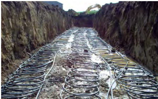
(c) Closed horizontal loop field
