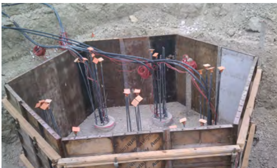
Figure 6-2 Energy piles construction
