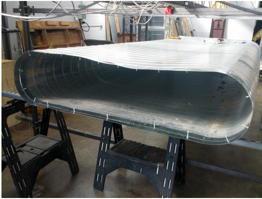
(a) Installing Coupling on First Duct Section
