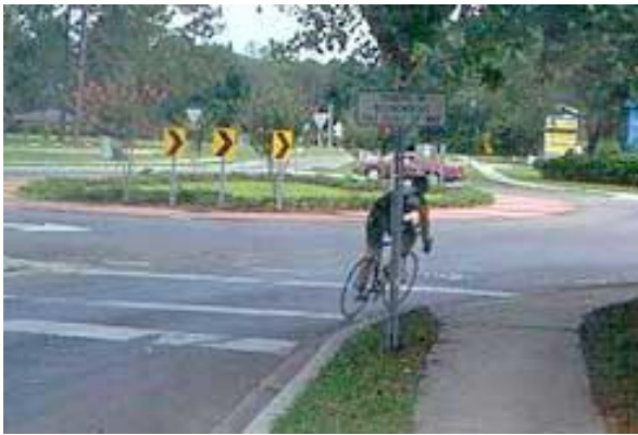
Figure 37. Example of a traffic roundabout. Source: Google.
