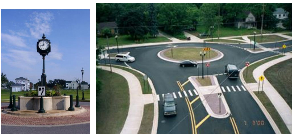
Figure 25. Example roundabouts. Source: Google.
