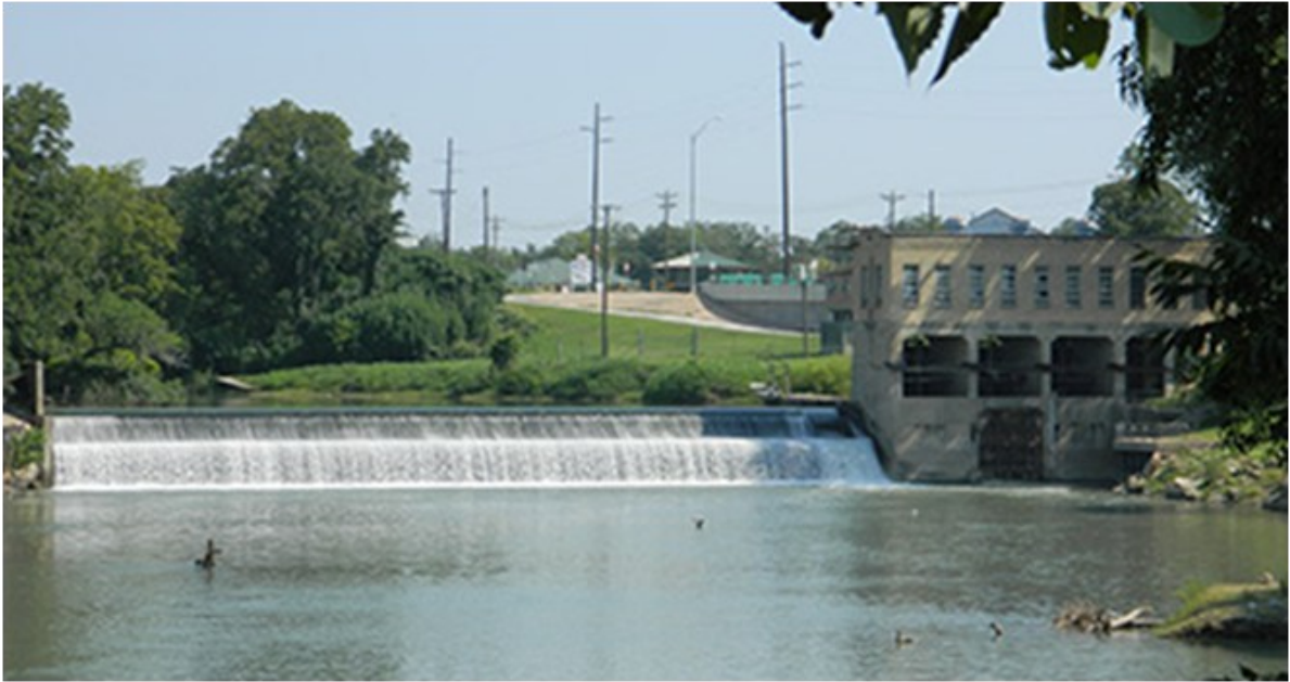
Figure 6.2: Water plant in Gonzales, Texas
