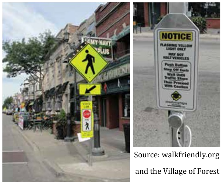
Figure 5.6: A solar powered pedestrian crosswalk signal.
