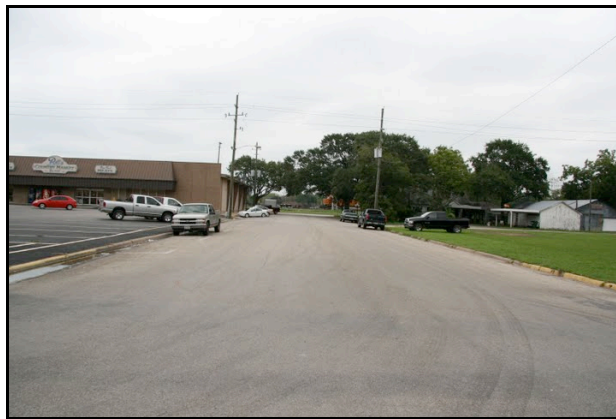
Figure 1.9 Fourth Street without sidewalks on both sides of the road
