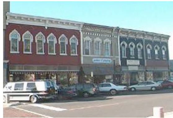
Example of consistent design elements. Vertical windows aligned on 2 nd floor with similar patterns and shape, and aligned cornices.
