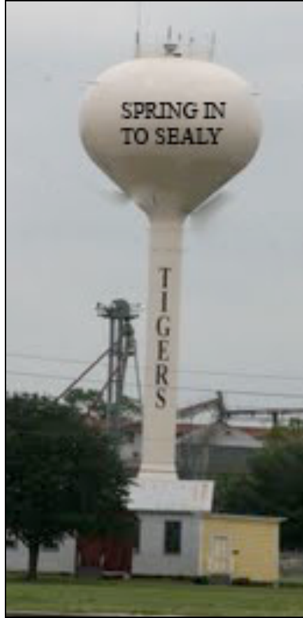
Figure 5.8 Example of a possible update to water tower for long-range landmark
