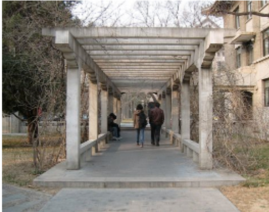
A covered walkway built to human scale with the roof close to the average height of a person using it
