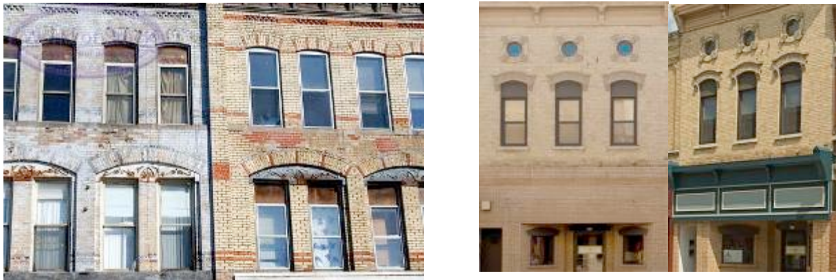
Examples of second story window preservation and uniformity
