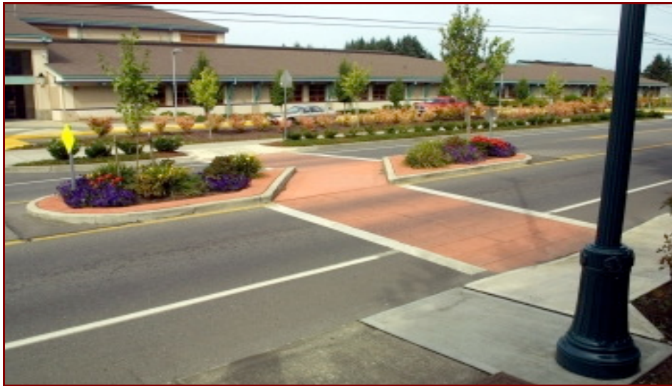
Figure 2.6 Zig-zag paved crosswalk design
