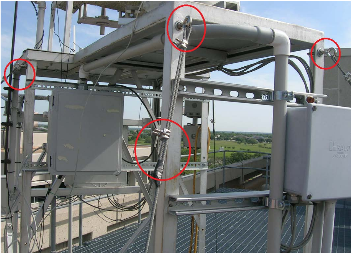
Figure 249 Securing of solar test bench
